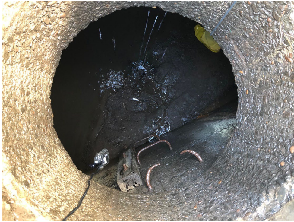
Photographs 18 (above) and 19 (below): View of bottom of sewer manhole MH-40 and sediment accumulation during 2/13/19 inspection
