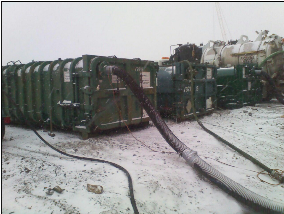
Photograph 9: View of vacuum boxes and vacuum truck during remediation of MH-40
