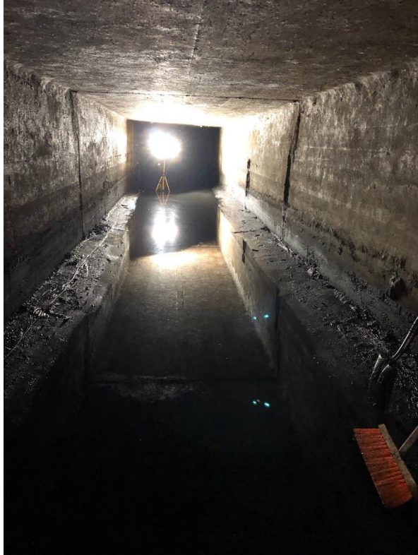
Photograph 2: Sewer after cleaning
