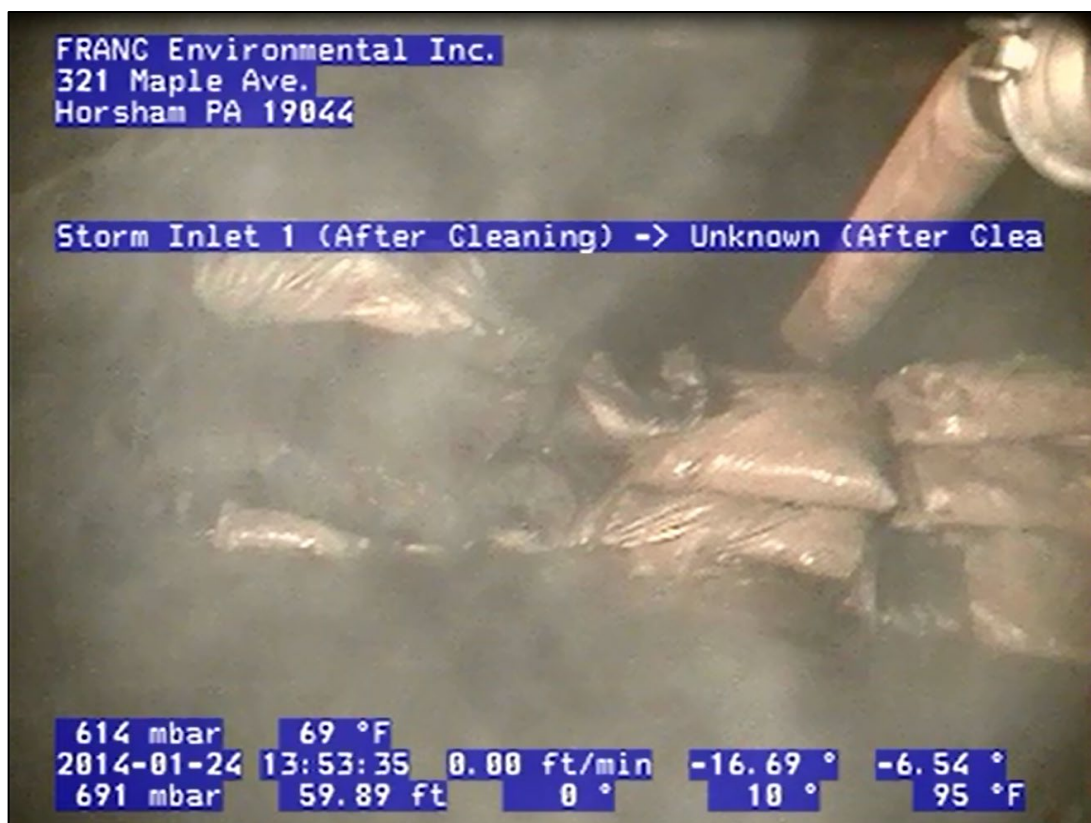
Photograph 14: View of newly constructed weir located eight feet downstream of MH-40 surface grate January 24, 2014
