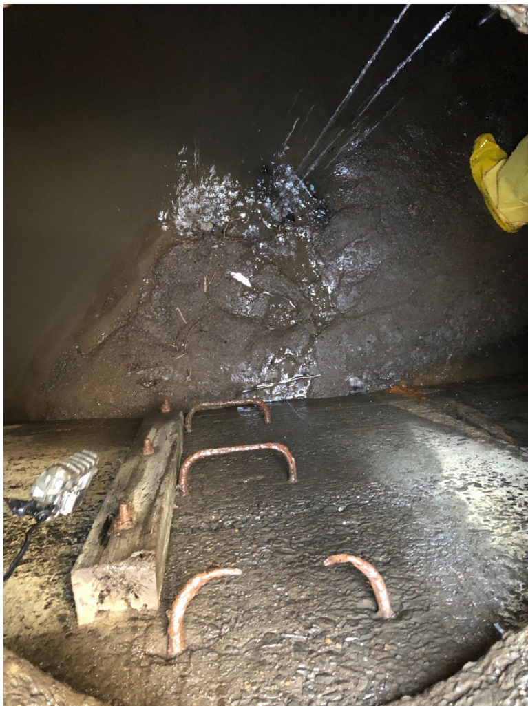
Photographs 18 (above) and 19 (below): View of bottom of sewer manhole MH-40 and sediment accumulation during 2/13/19 inspection
