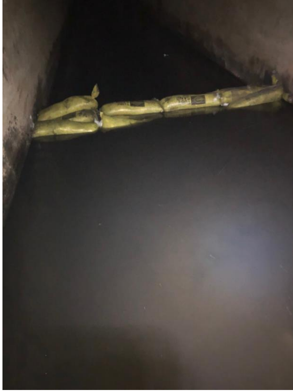
Photograph 1: Sewer structure with weir
