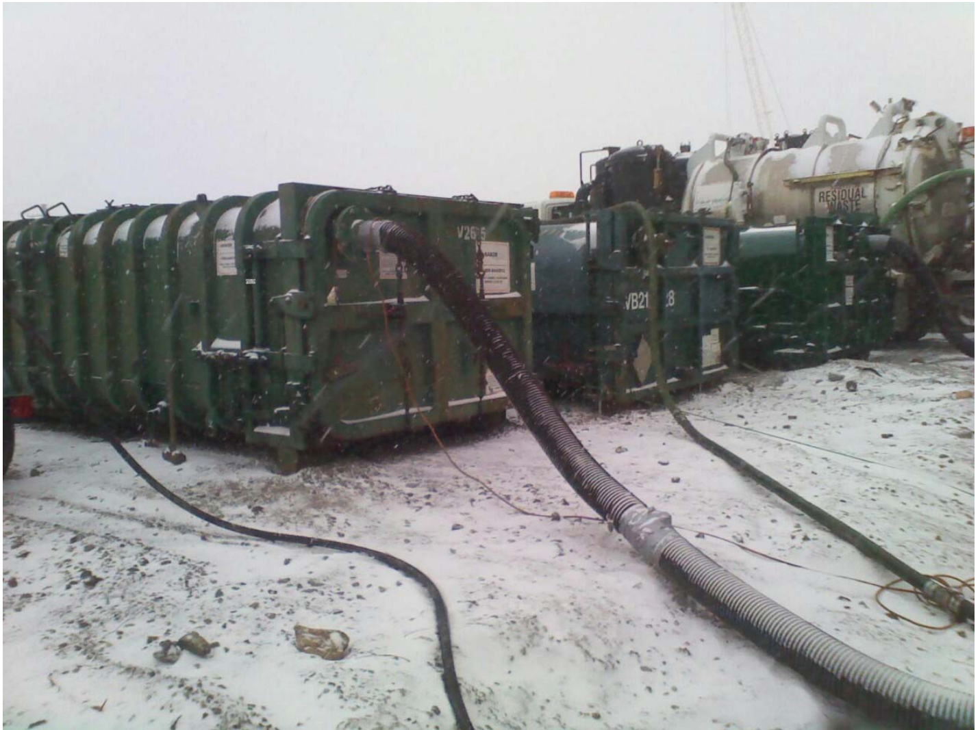
Photo 1. View of Vacuum Box during sediment removal.
