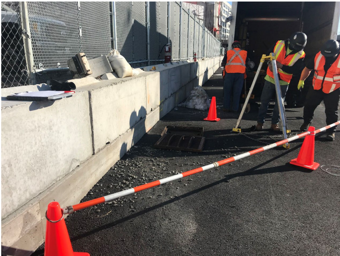
Photographs 23 (above) and 24 (below): View of sewer manhole MH-40 at grade and confined space entry during 2/26/21 inspection
