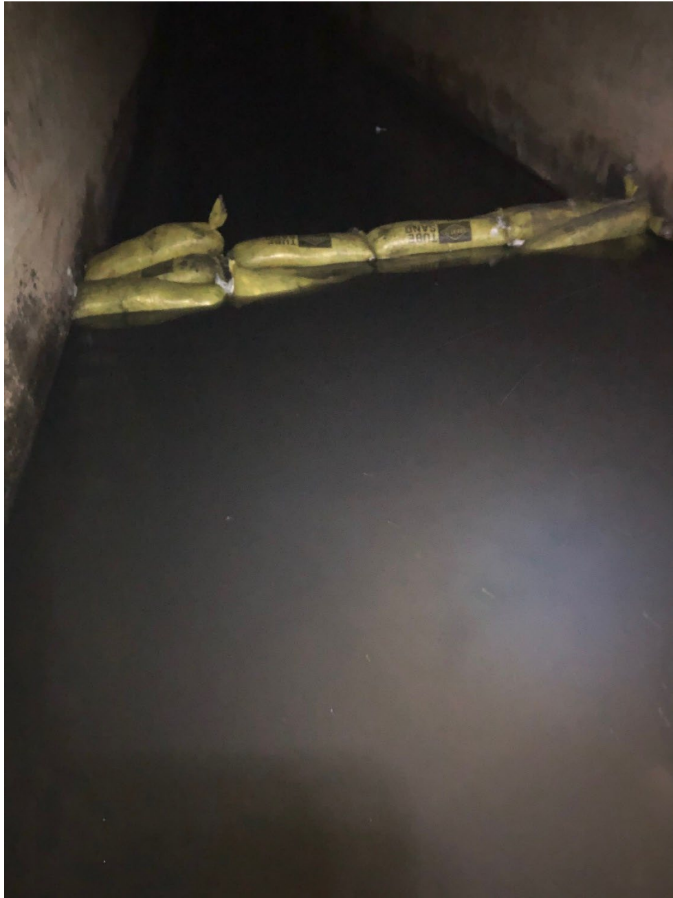
Photograph 22: View of newly constructed weir located eight feet downstream of MH-40 surface grate during November 2020 (by MTA)
