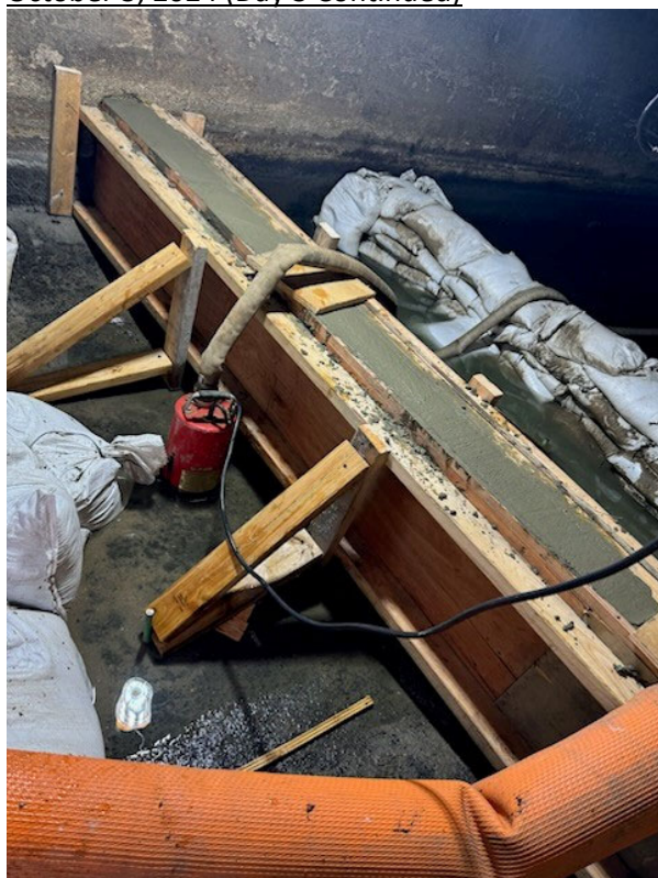
Contractor (KNR) poured the concrete weir wall.
