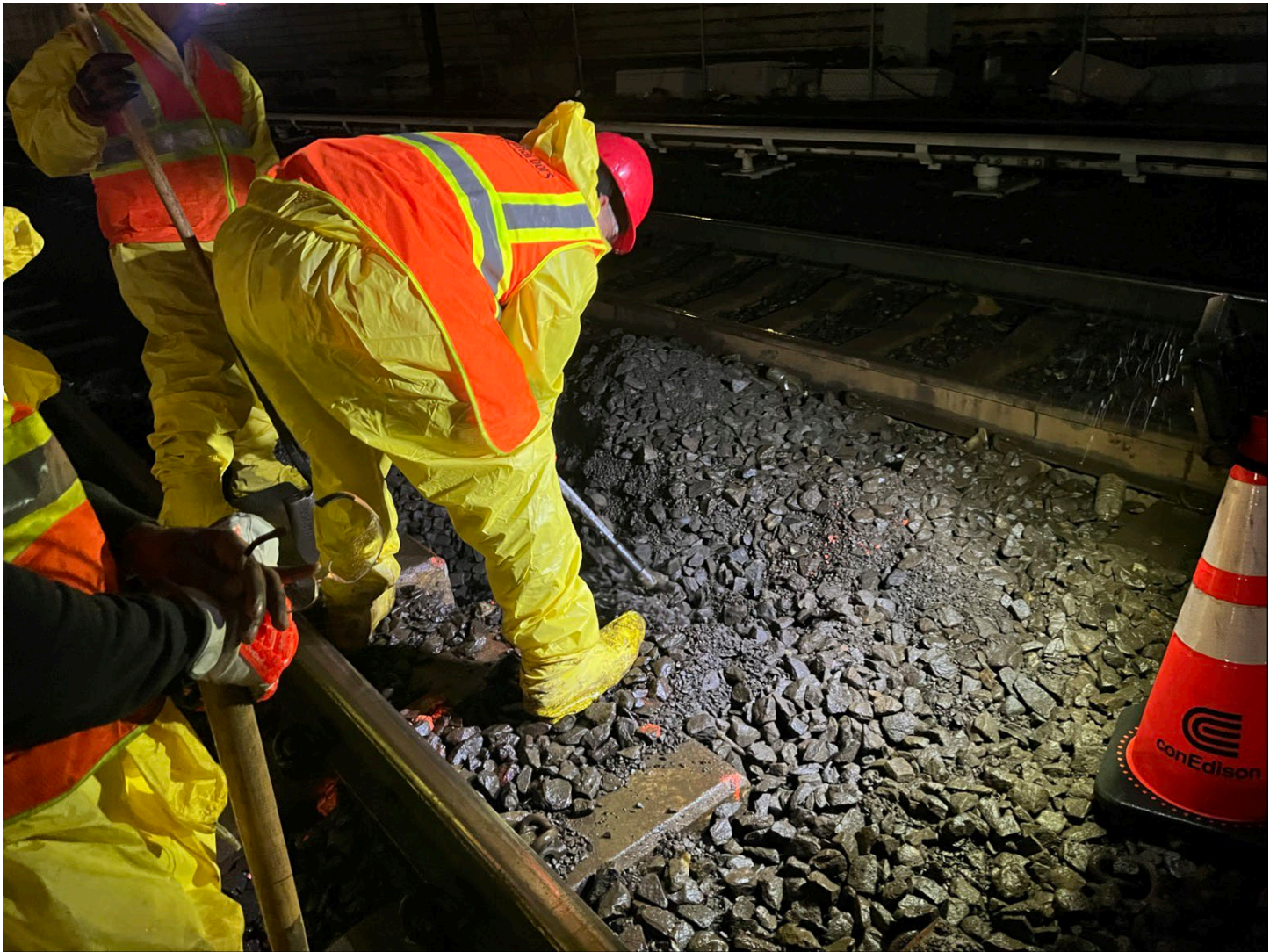
Photo 4: View facing northeast; Amtrak laborers backfilling holes after collecting samples.
