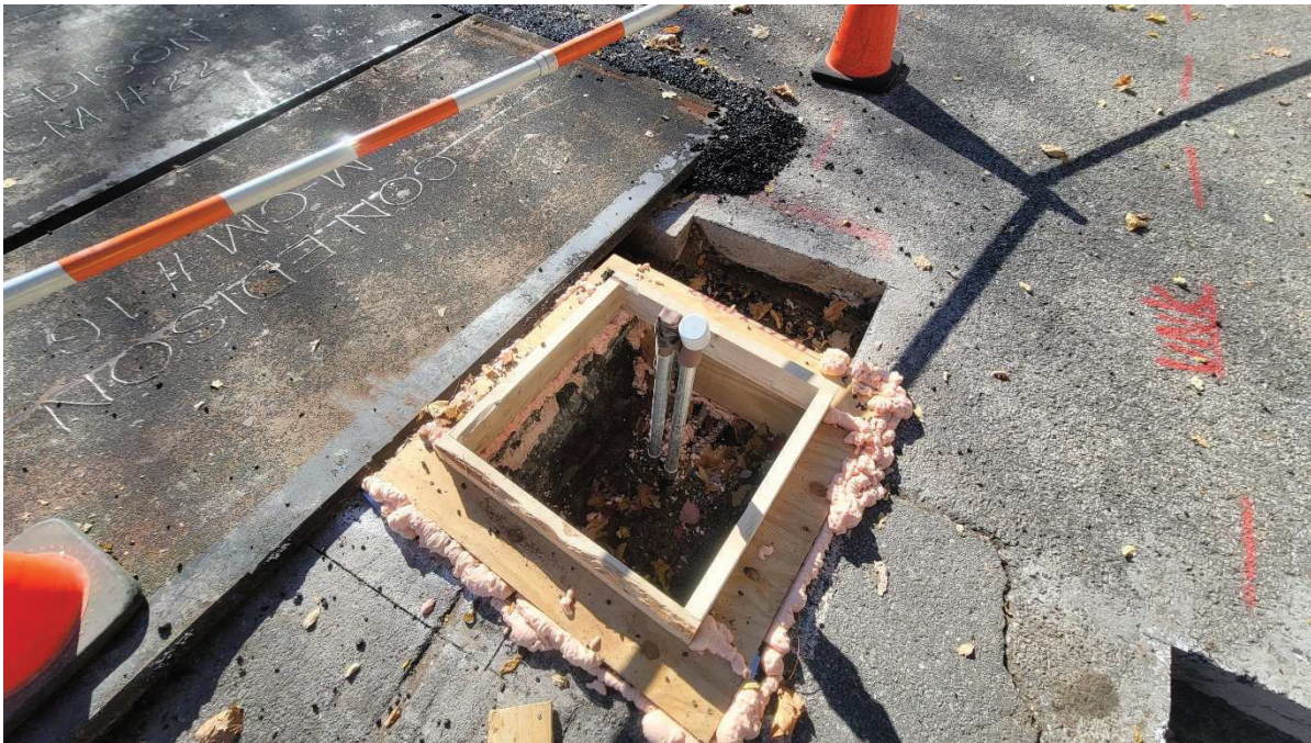
Day 5, Construction crew and other have created wooden frames for Grouting and filled the trenches with soil
