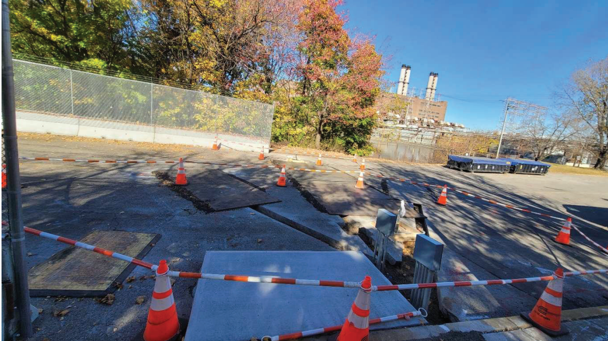
Day 5, Construction crew and other have created wooden frames for Grouting and filled the trenches with soil
