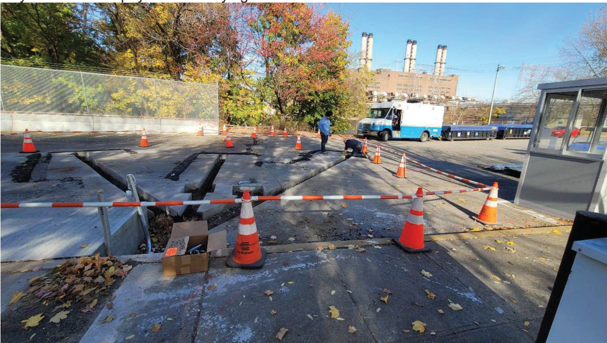
Day 4 shows the electrical crew laying conduit pipes.
