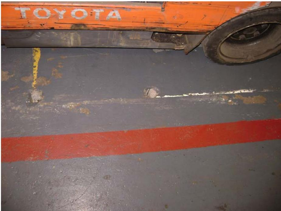
Photo #90: Holes in subslab.
