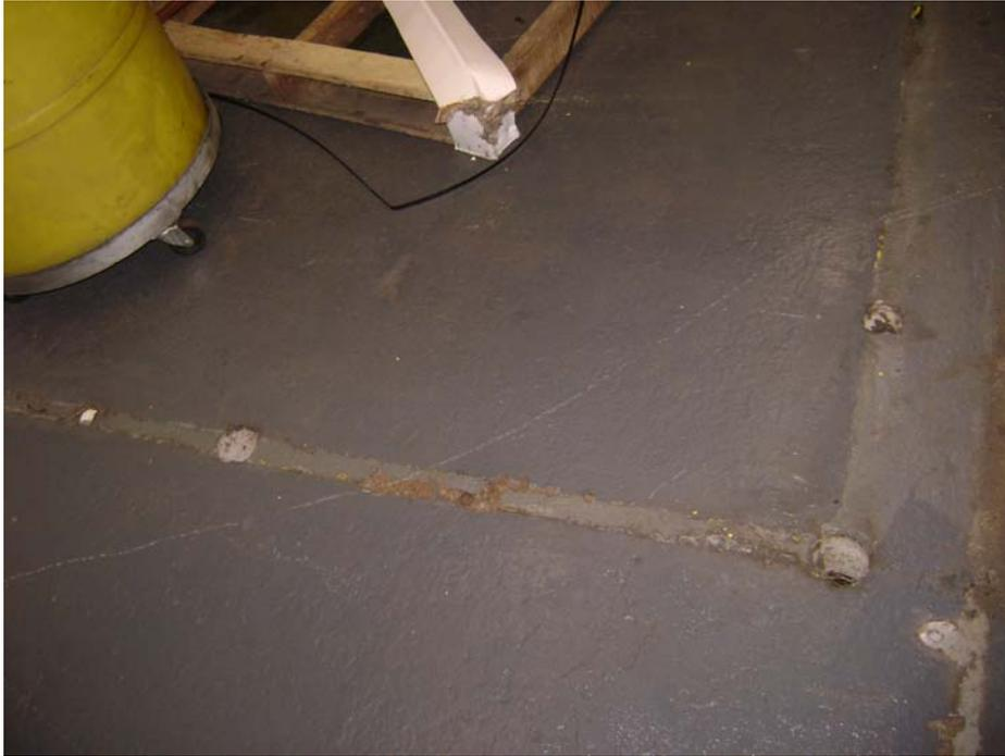
**Photo #87: Holes in subslab where heavy equipment were previously bolted in. The openings penetrate through the subslab.**
