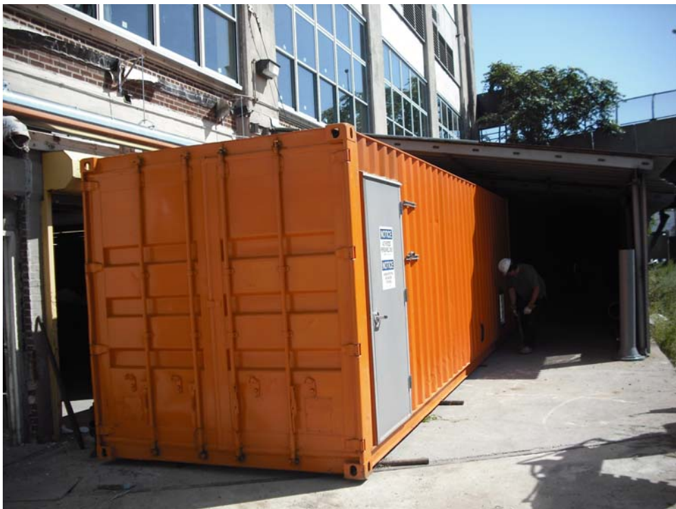
Photo 4: Extraction system skid being transported to underneath cover
