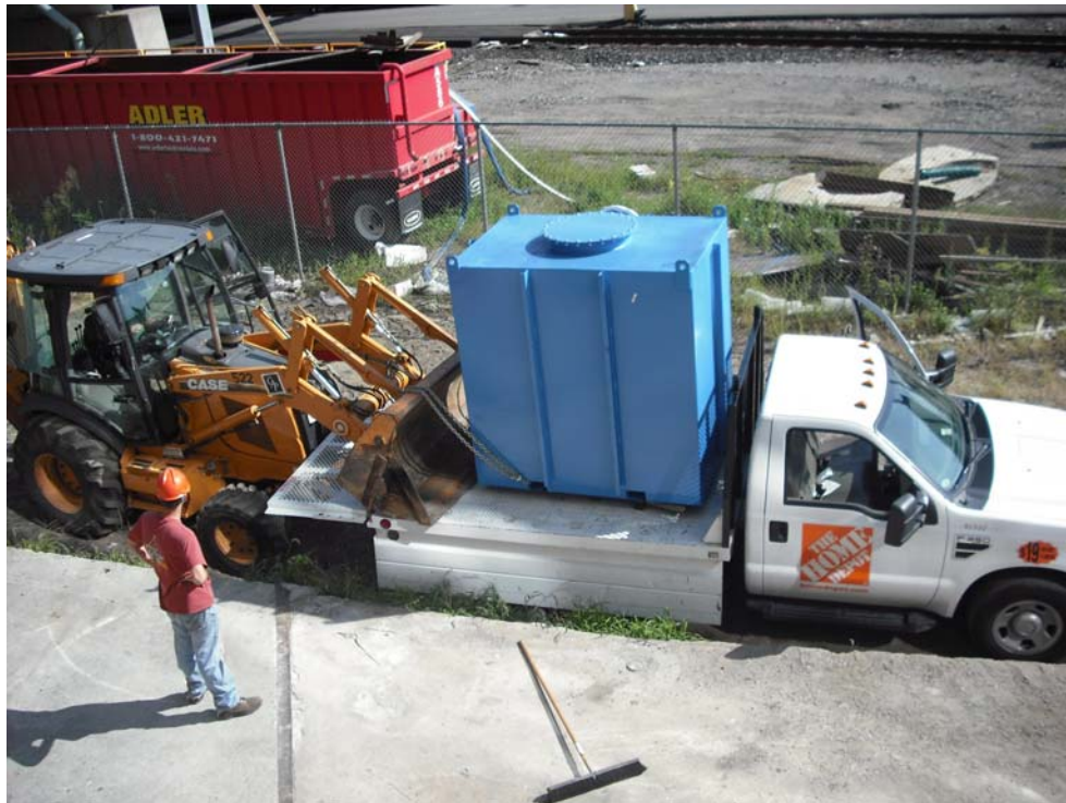
Photo 5: Delivery of vapor phase granulated activated carbon unit
