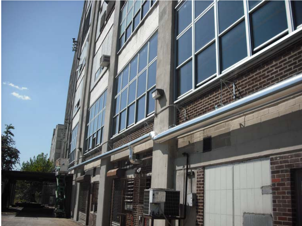
Photo 3: Exterior pipe with insulation and aluminum cover
