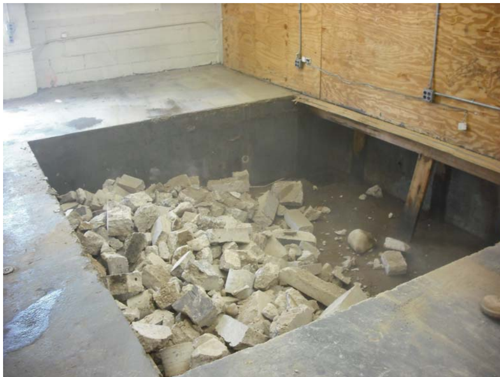
Photo 6: Concrete cuttings placed into equipment vault prior to pouring of new concrete
