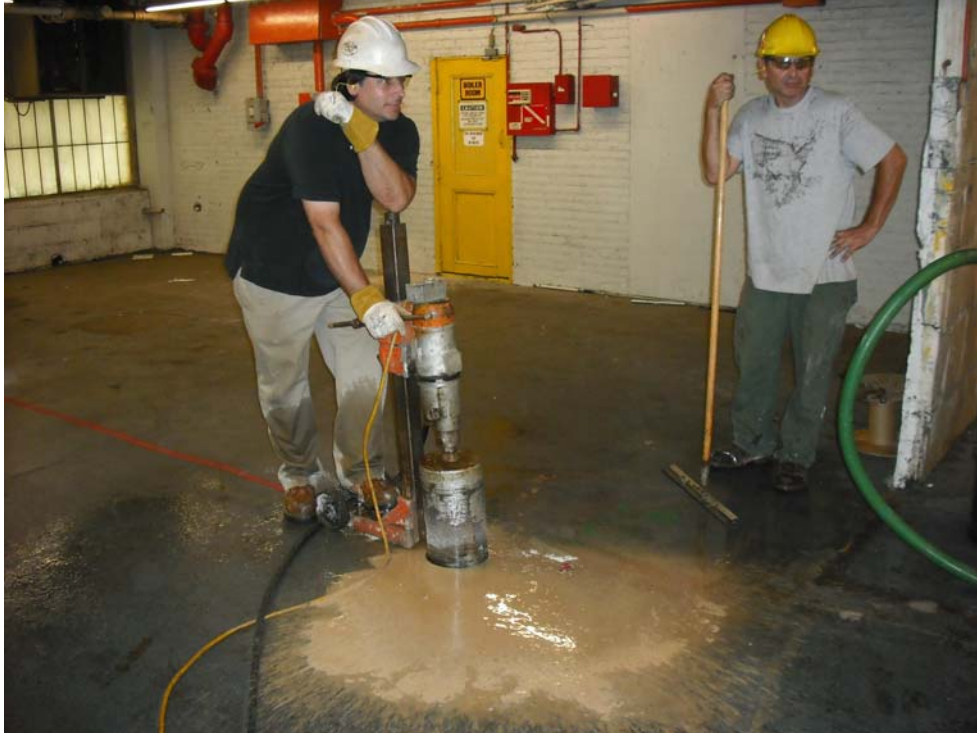
Photo 1: Crew coring for installation of extraction sump
