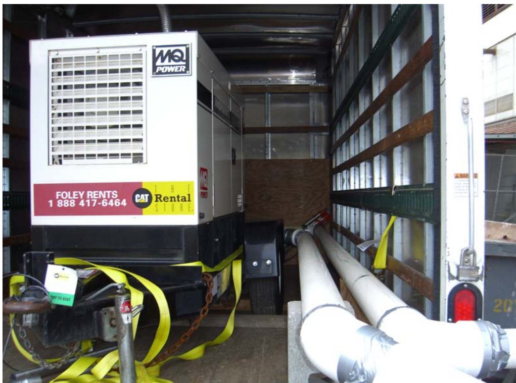
Photo 2: Blower Influent and Effluent
