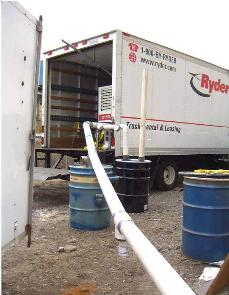
Photo 3: Vapor Piping and VPGAC Adsorber
