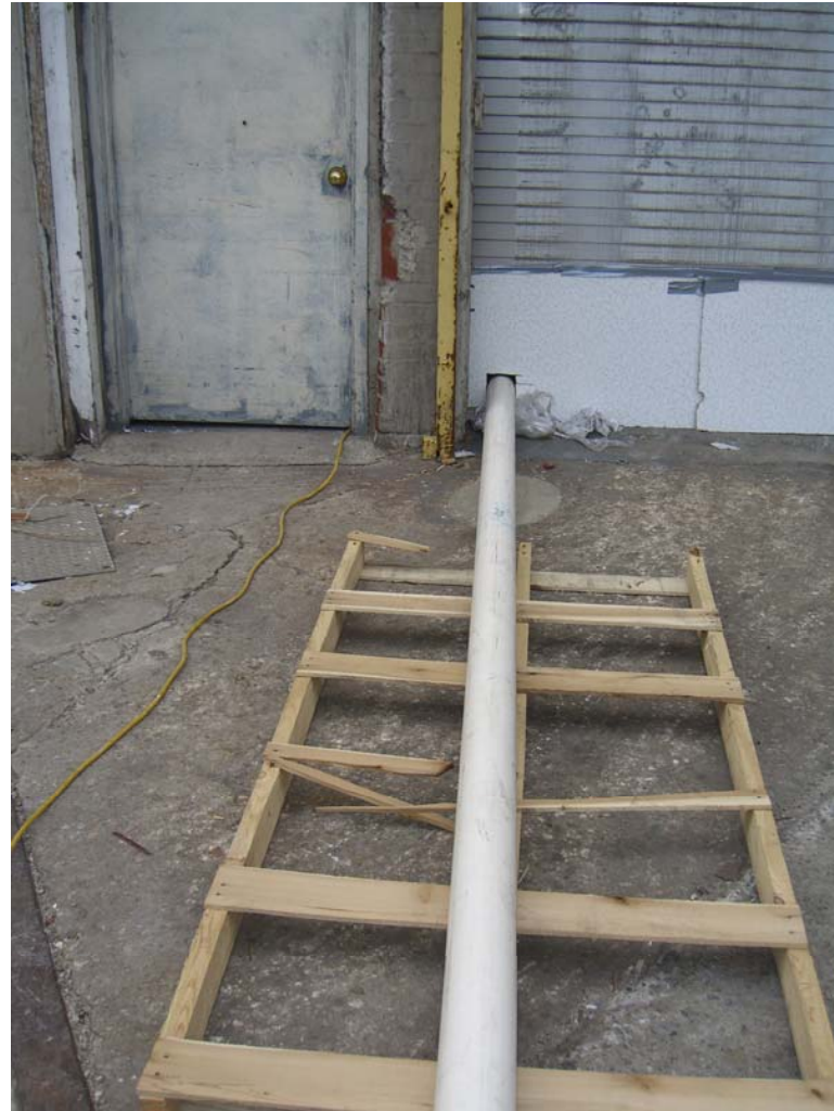
Photo 6: Pipe Penetration from Outside
