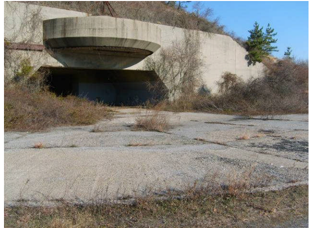
Photo E.4 – Battery Harris West.
