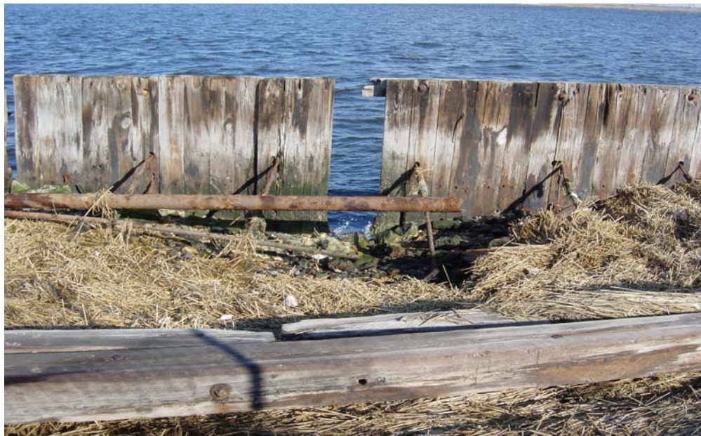
Damage to the Bulkhead has resulted in debris washing on the beach during high tide.
