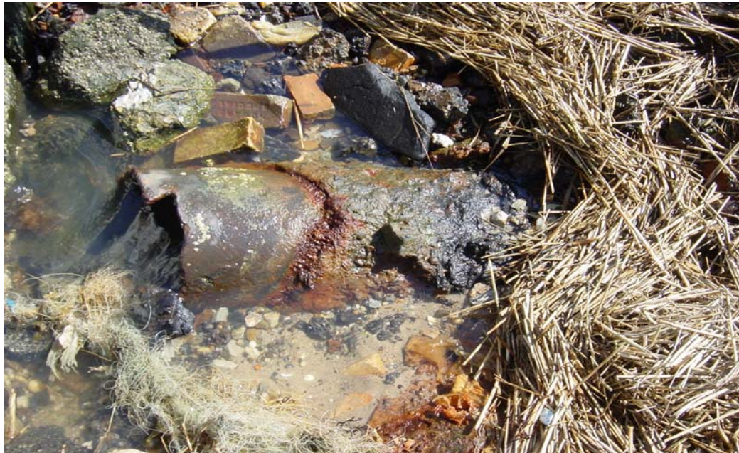
The 12-inch diameter pipe. A section of soil measuring approximately 3 feet X 3 feet was excavated by hand. The pipe was inspected and sealed with Portland Cement to prevent future exposure pathways.
