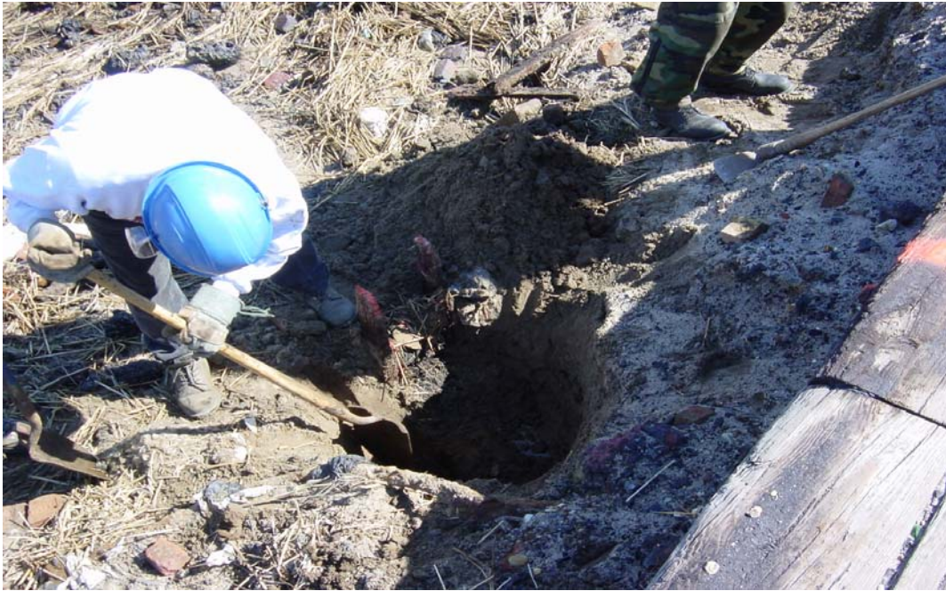
Coastal Environmental manually excavated the soil to reach the pipes located beneath the ground surface.
