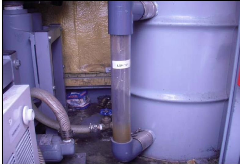
Picture 001.jpg - Knock out water was drained from both systems into a 55-gallon drum.
