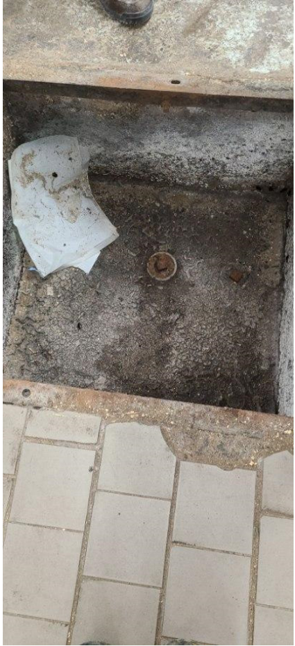
Inside one of the vaults/cleanout.
