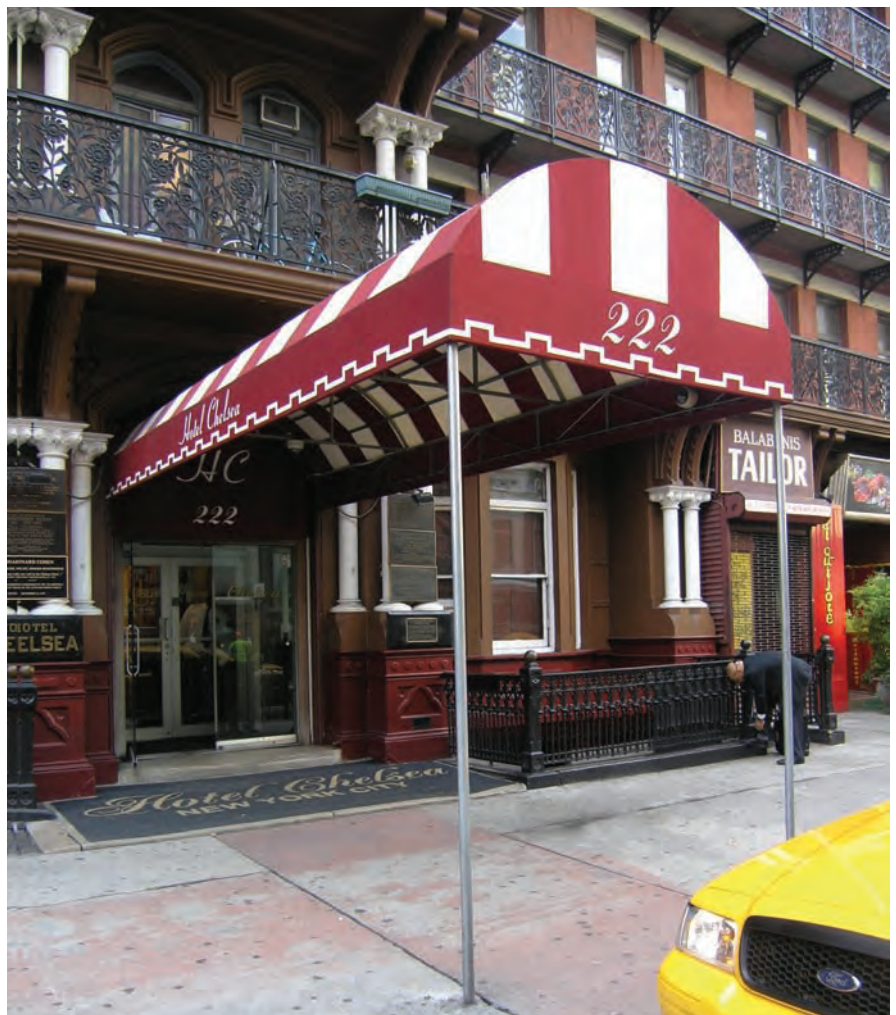
NYC DOT authorization is required before installing a canopy over the sidewalk.
