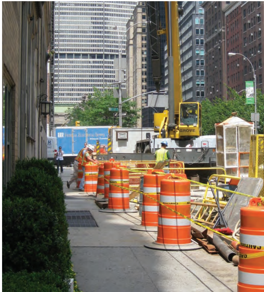
Crane placed on the street for construction activity. Cranes may require permits from DOB in addition to NYC DOT.
