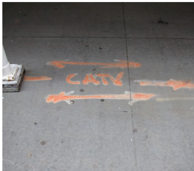
It is essential to call New York 811 before digging anywhere, including sidewalks and soil. This New York 811 marking shows where a cable television line is located beneath the sidewalk.
