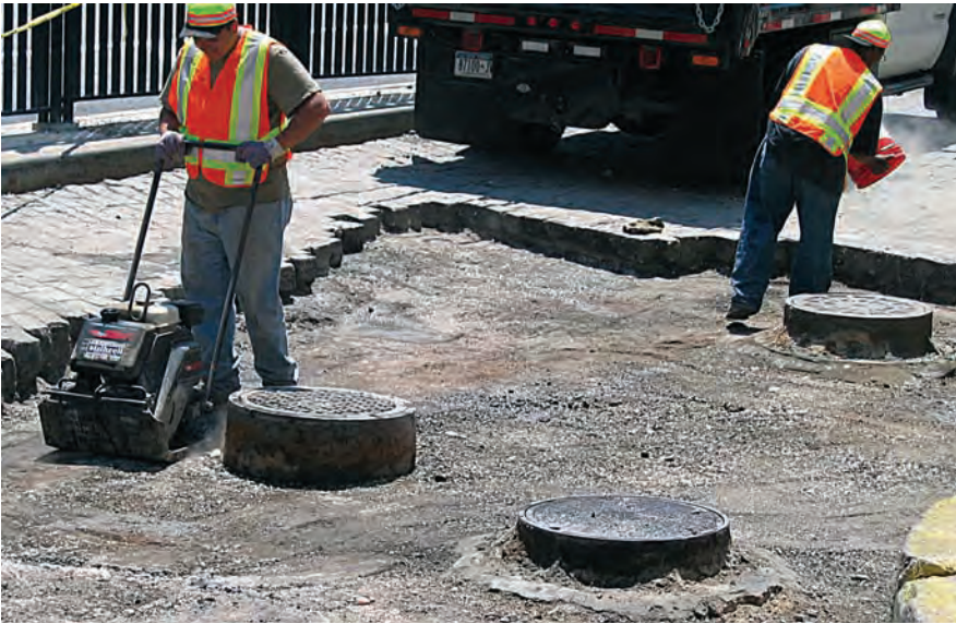
NYC DOT coordinates street opening and other construction on streets.
