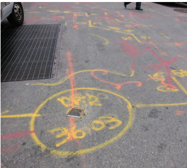
Streets can hide a complex infrastructure of underground utilities. One call to New York 811 provides for where gas (yellow), electric (red) and phone (orange) are located.
