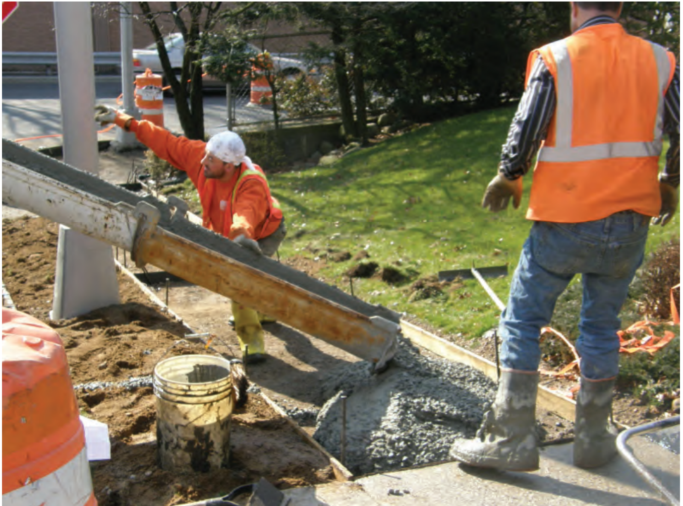
Workers pour cement during sidewalk reconstruction.
