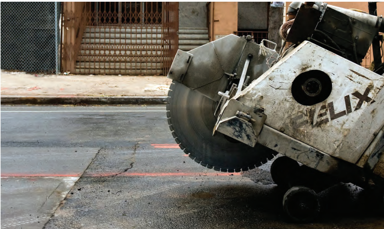
Coordination aims to reduce street excavation work on recently repaved streets.
