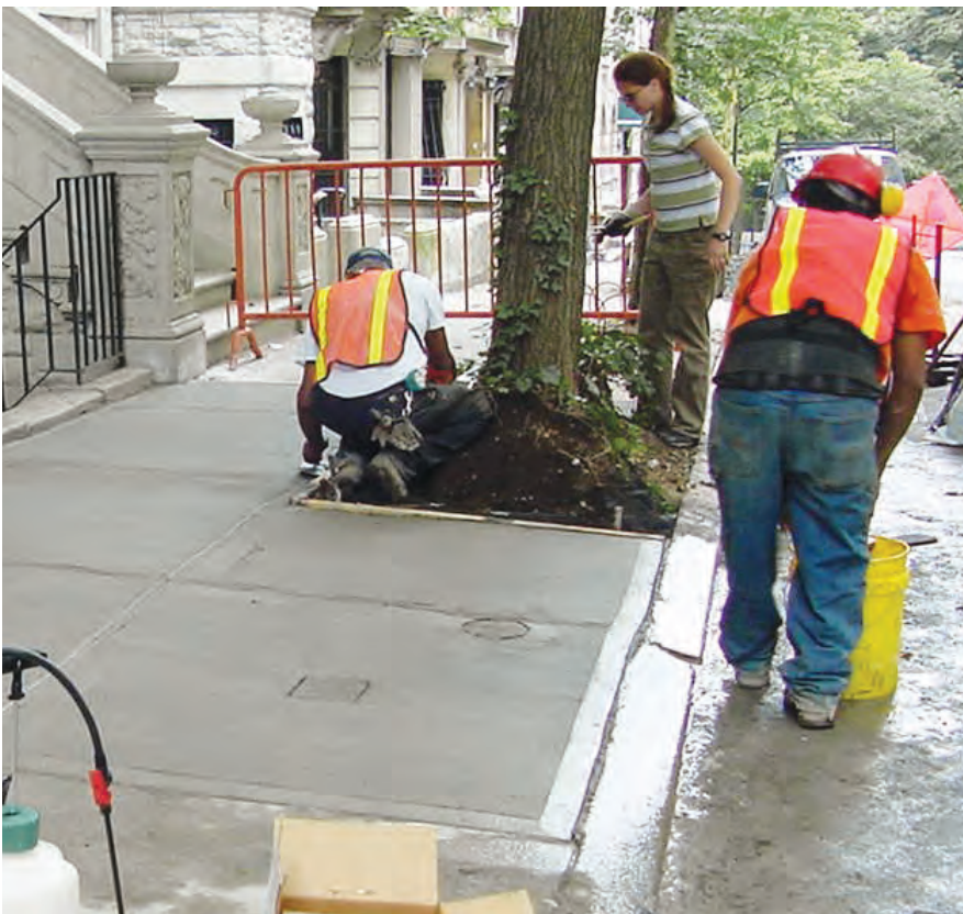
A temporary sidewalk closure while a sidewalk repair is underway.
