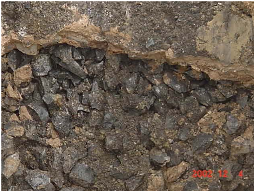
Test Trench showing Gas Holder Foundation and Sub Base
