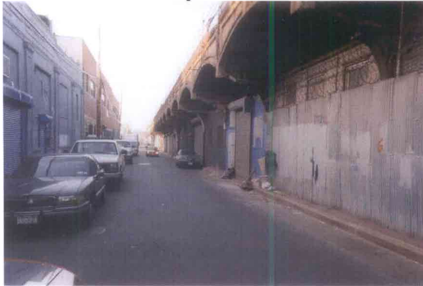
100 th St (looking South down 100 th Street – Site Bays on the right)
