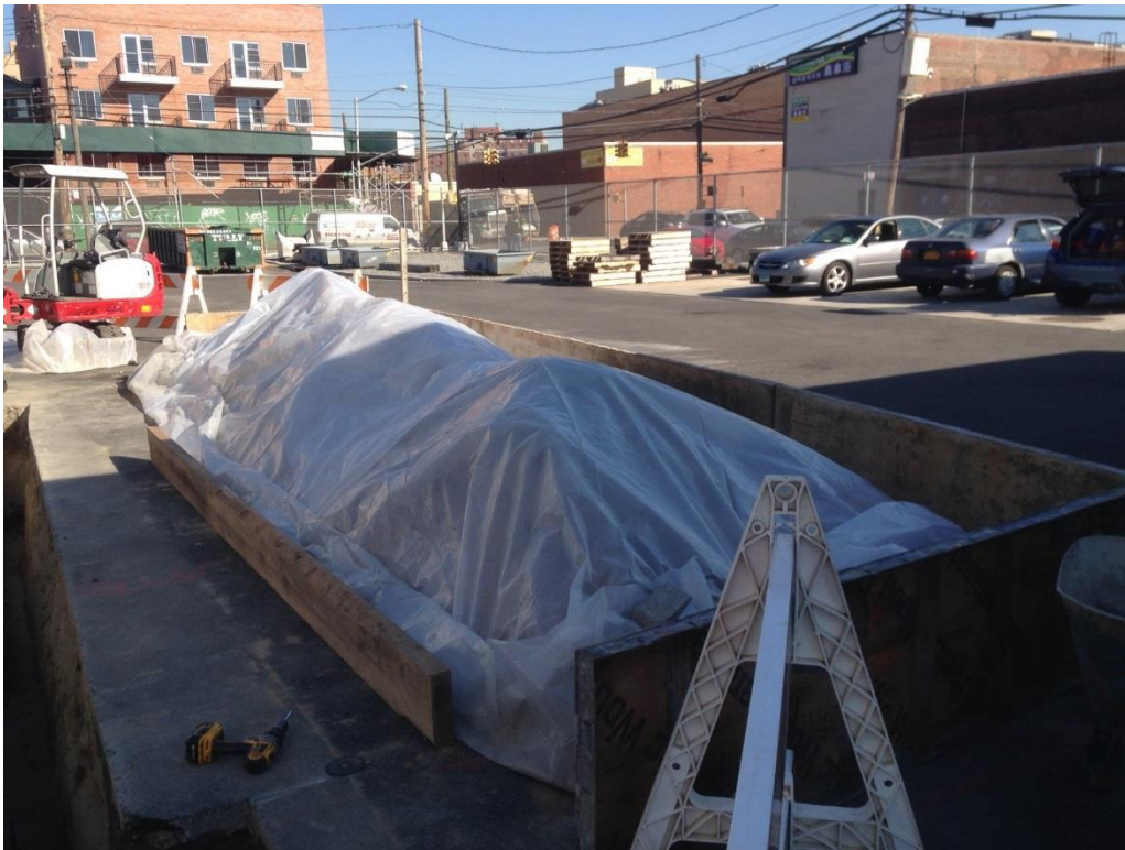
Photo 10: Excavated soil managed with appropriate containment (Facing Southeast)
