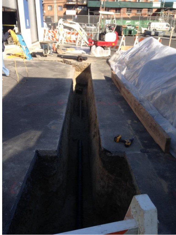
Photo 9: View of open drain pipe trench excavation (Facing East)
