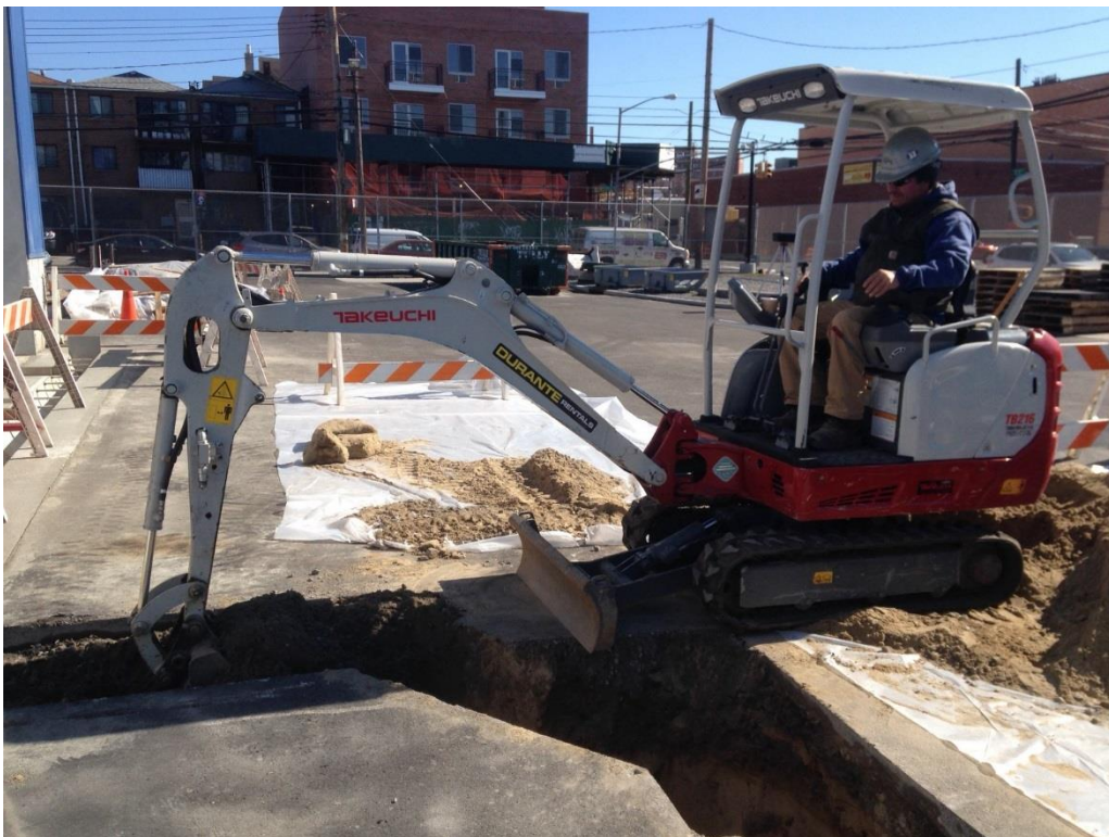
Photo 8: Excavation of the drain pipe trench with an excavator (Facing East)
