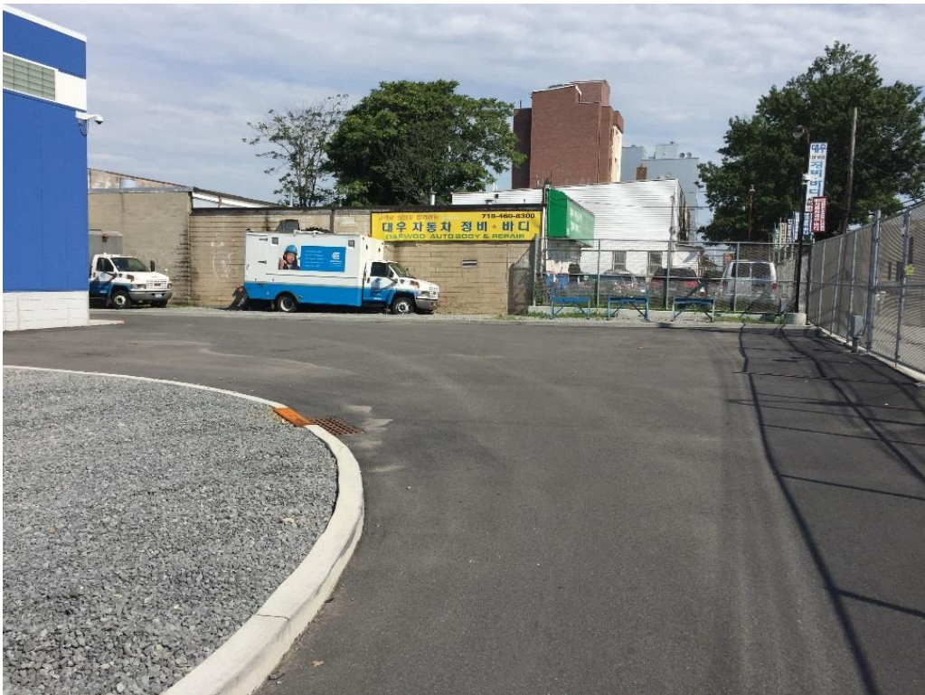
Photo 6: New Flush-truck facility driveway (Facing North)
