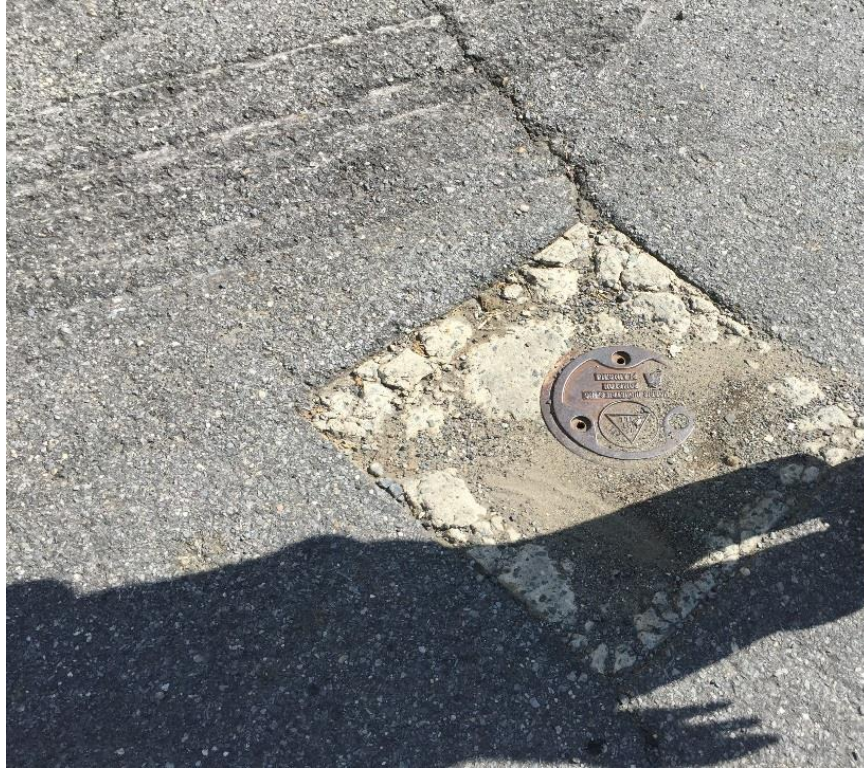
Photo 1: Monitoring Well MW-6 (Facing Northeast)
