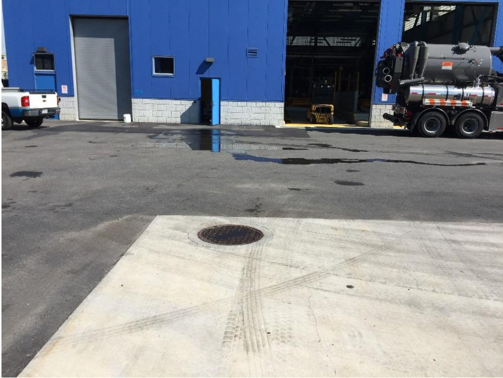
Photo 5: New Flush-truck facility (Facing North)
