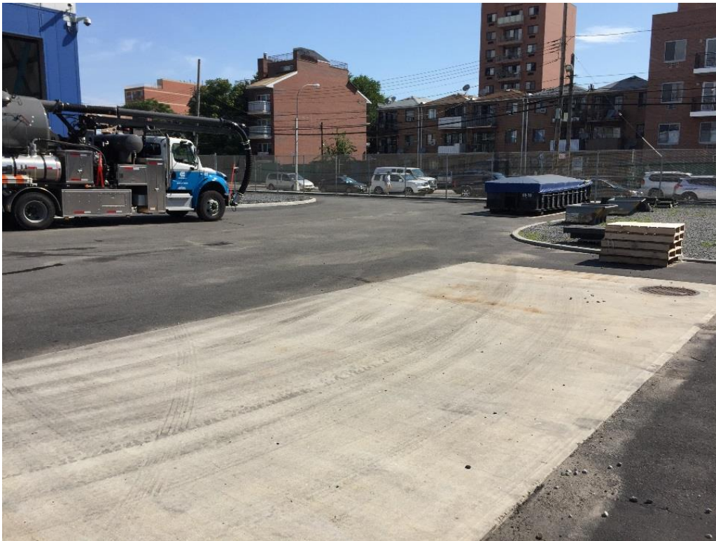
Photo 4: New Flush-truck facility driveway (Facing Northeast)
