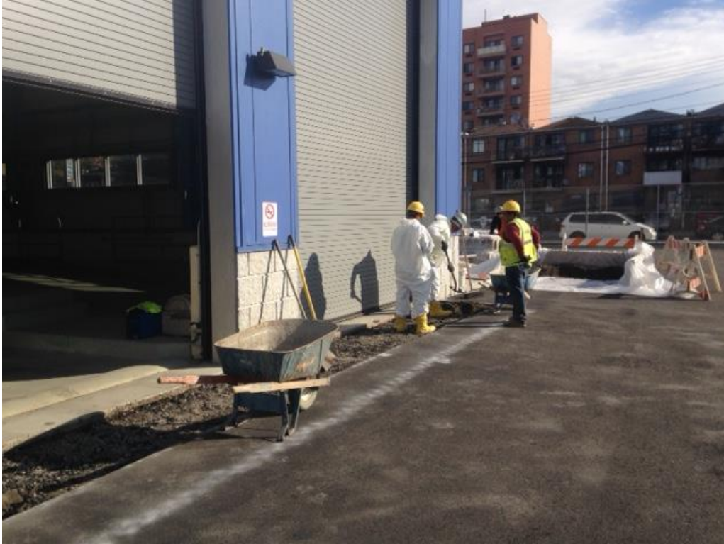
Photo 7: Start of ground disturbance with asphalt removal (Facing Northeast)
