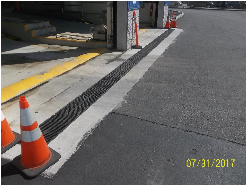
Photo 10: Trench drain installed and excavation back filled and capped (Facing East)
