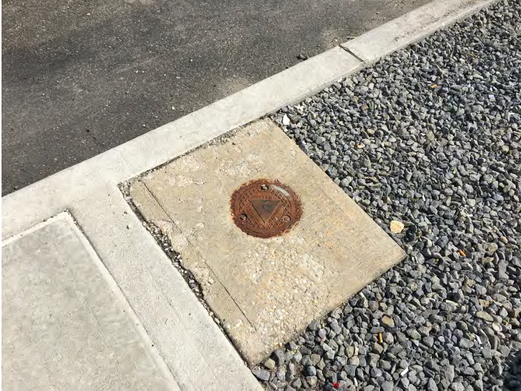
Photo 3: Monitoring Well MW-13 (Facing North East)
