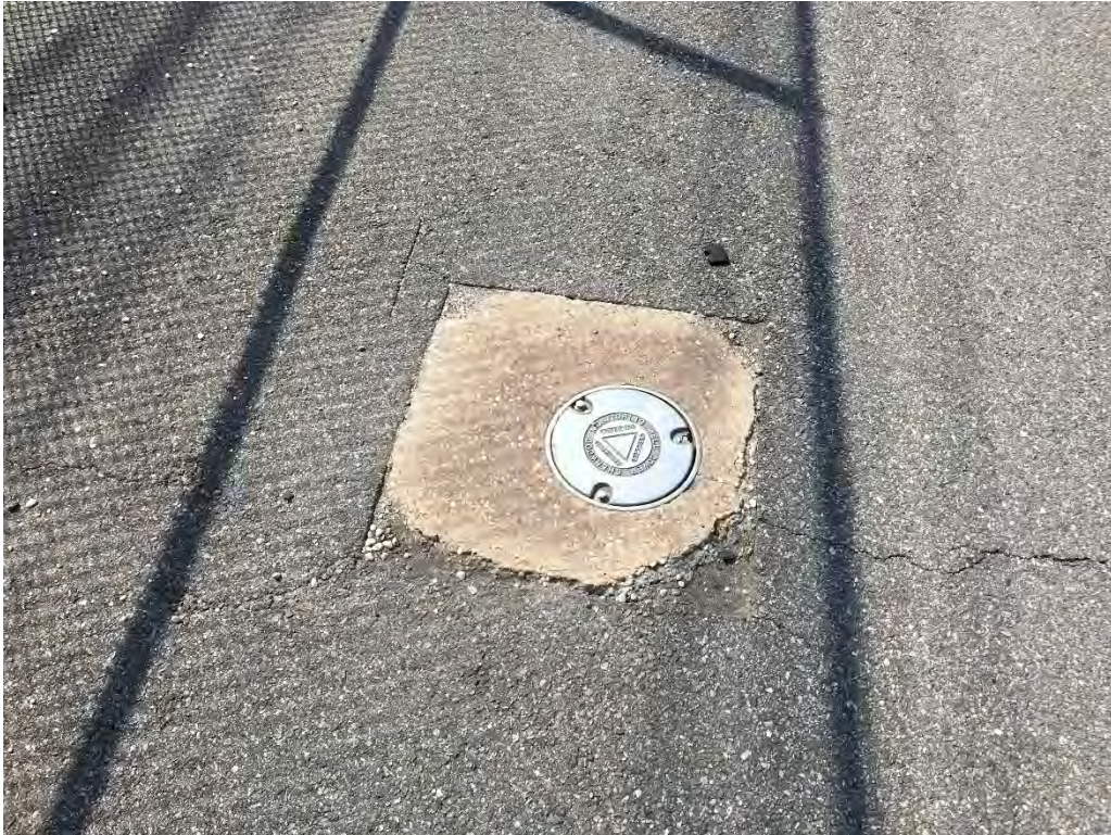
Photo 4: Monitoring Well MW-9 (Facing South)
