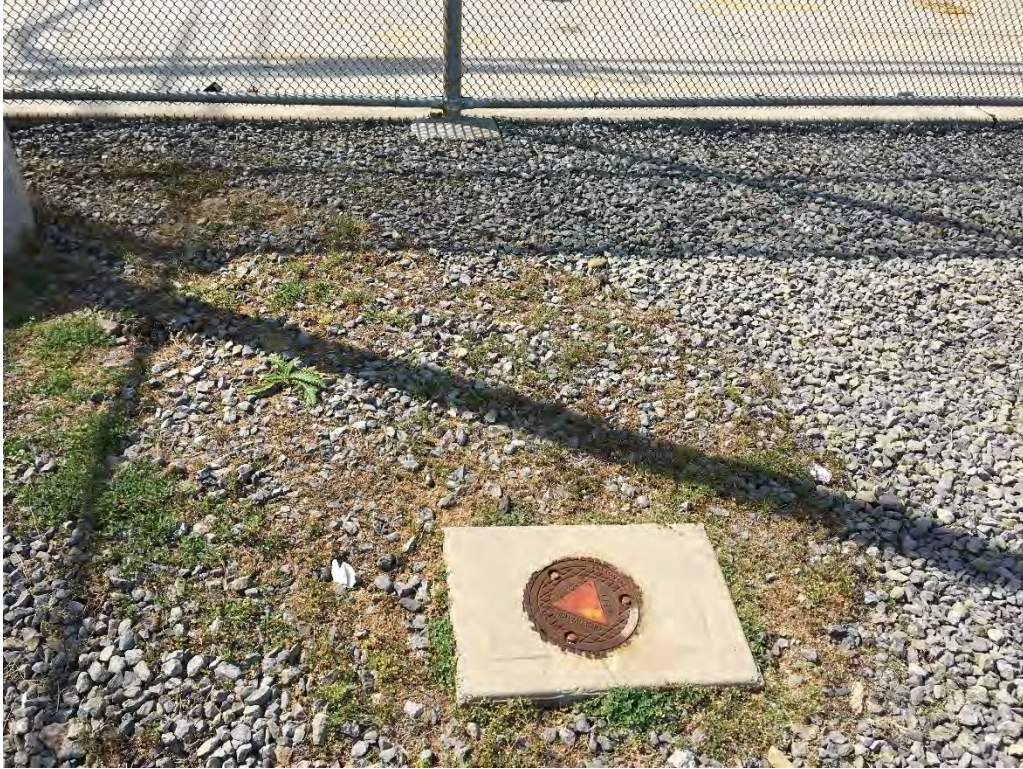
Photo 5: Monitoring Well MW-17 (Facing South)
