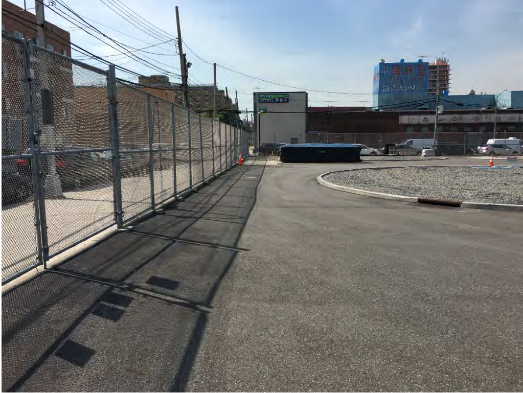
Photo 9: Perimeter Chain-link Fencing (Facing South)
