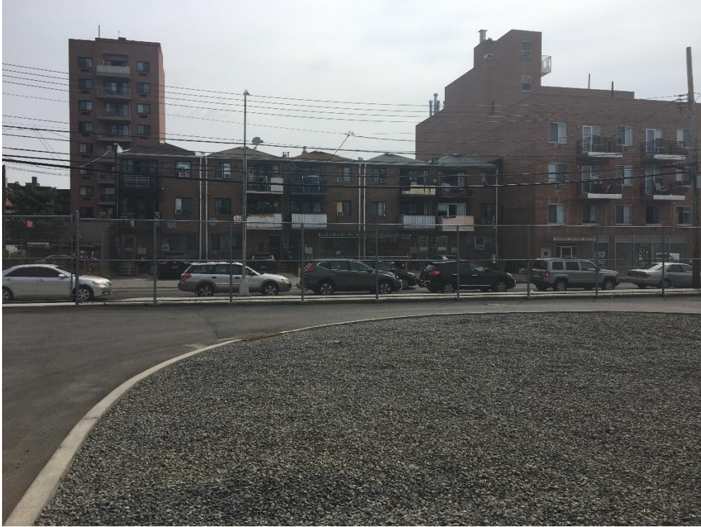
Photo 9: Perimeter Chain-link Fencing (Facing East)
