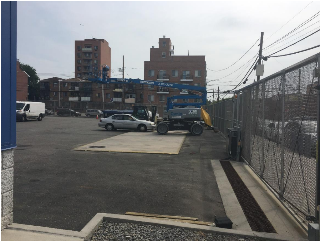
Photo 10: Perimeter Chain-link Fencing (Facing East)
