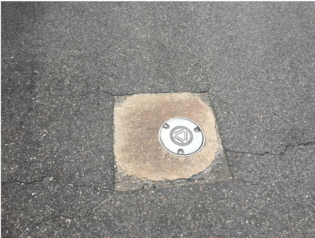
Photo 4: Monitoring Well MW-9 (Facing South)
