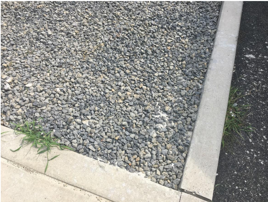
Photo 2: Location of Former Monitoring Well MW-14 (Facing East)
