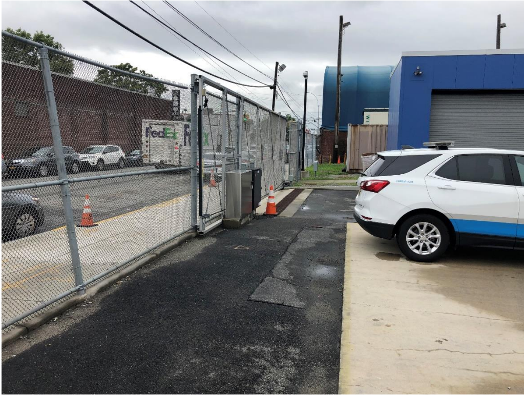
Photo 9: Perimeter Chain-link Fencing (Facing West)
