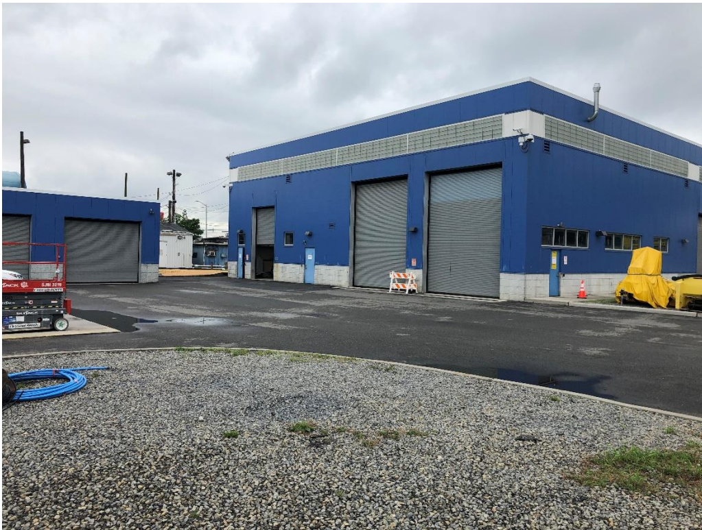
Photo 10: Flush Truck Facility (Facing Northwest)
