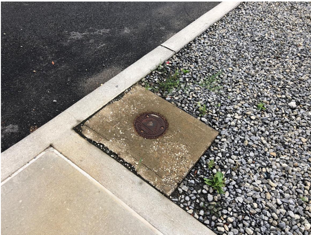
Photo 2: Monitoring Well MW-13 (Facing East)
