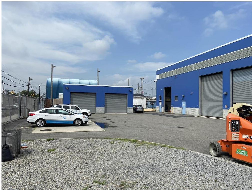
Photo 10: Flush Truck Facility (Facing Northwest)
