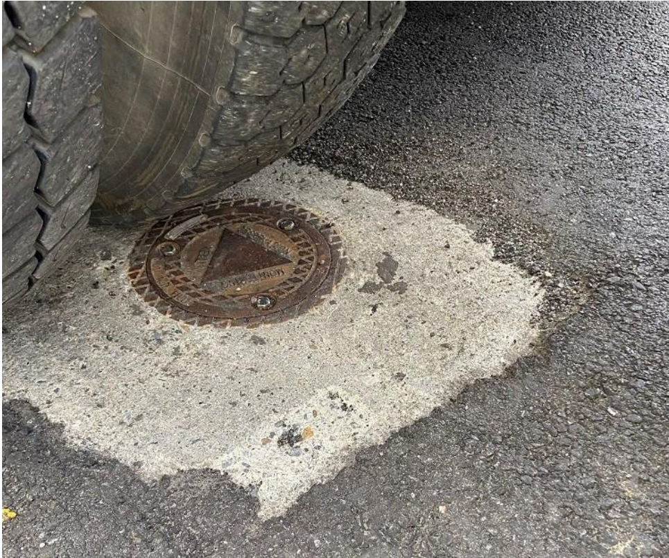
Photo 1: Monitoring Well MW-6 (Facing Southwest)
