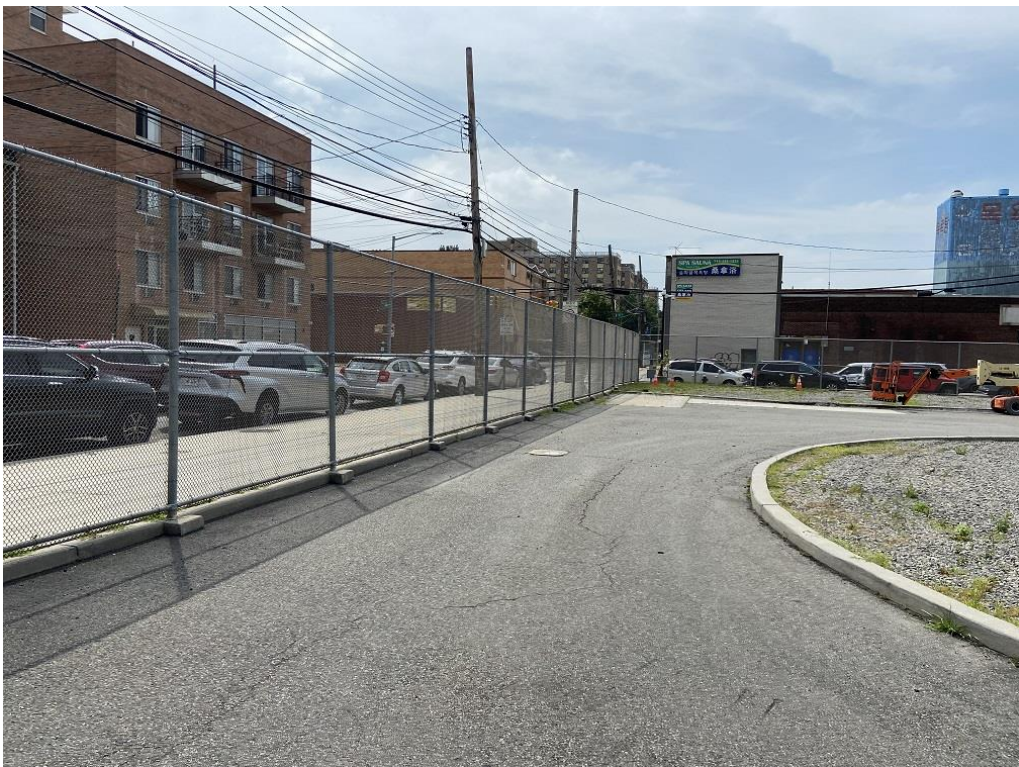
Photo 8: Perimeter Chain-link Fencing (Facing South)
