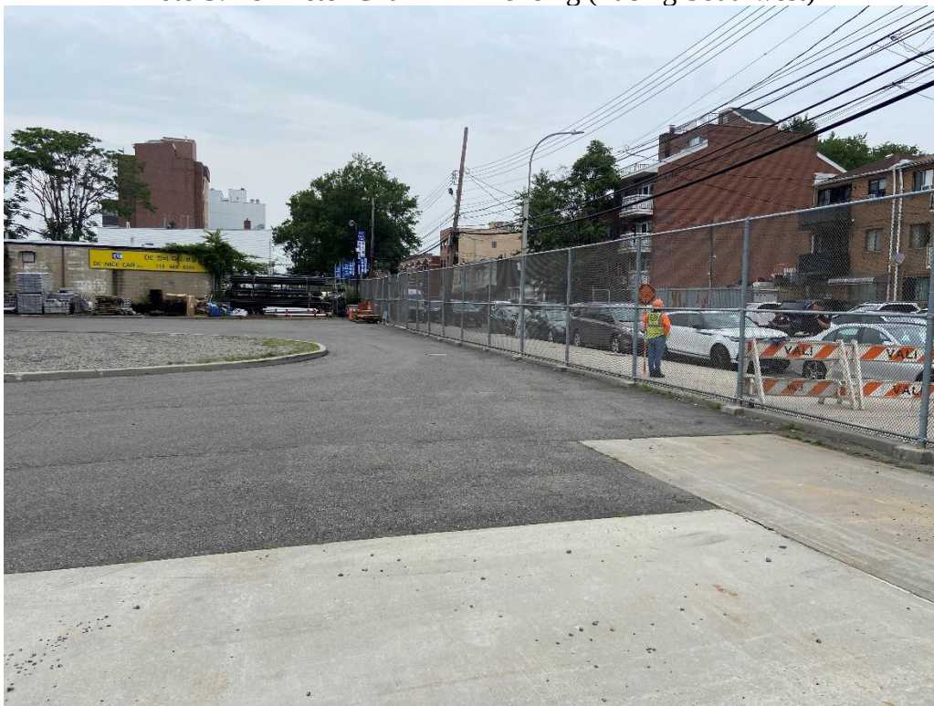
Photo 6: Perimeter Chain-link Fencing (Facing North)
