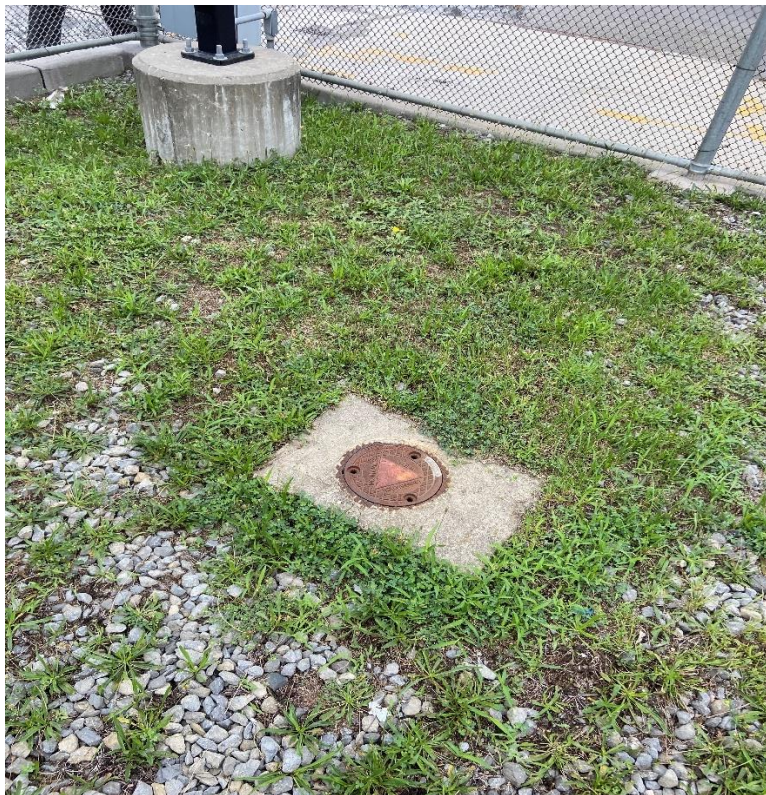
Photo 2: Monitoring Well MW-17 (Facing South)
