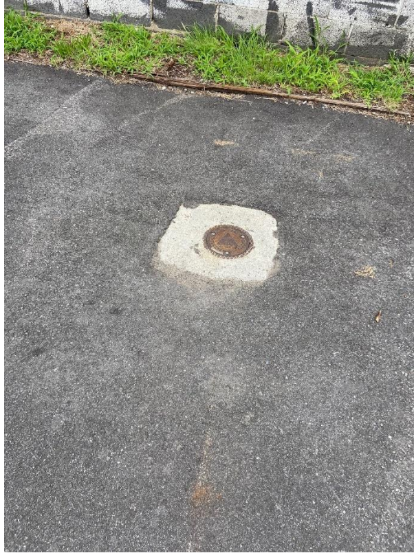
Photo 9: Flush Truck Facility (Facing Northeast)
