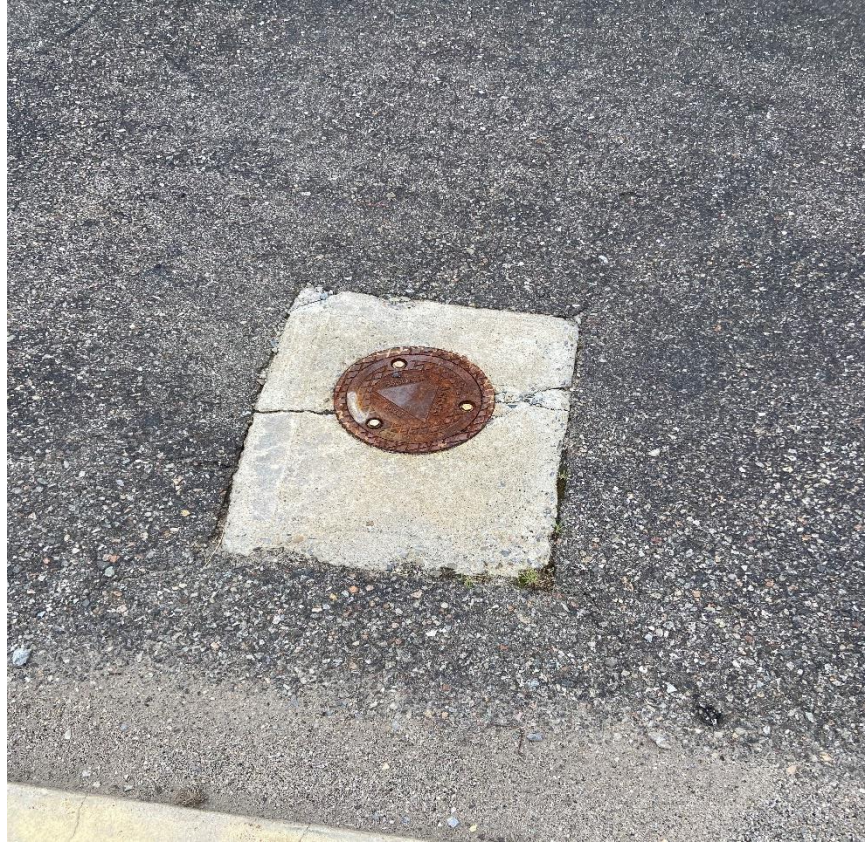
Photo 3: Monitoring Well MW-16 (Facing South)
