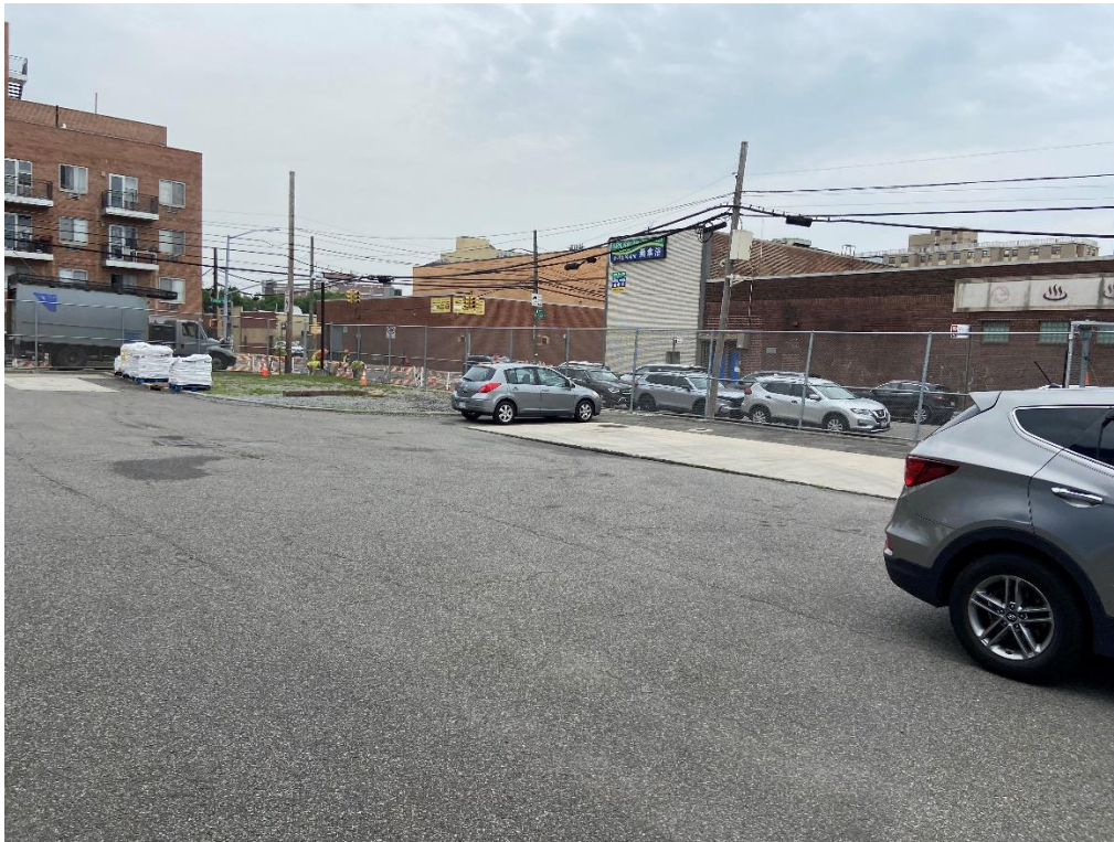
Photo 5: Perimeter Chain-link Fencing (Facing Southwest)
