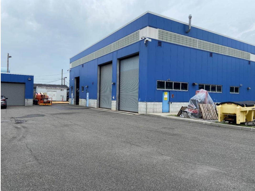
Photo 7: Flush Truck Facility (Facing Northwest)
