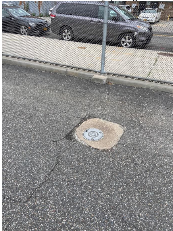
Photo 10: Flush Truck Facility (Facing Northeast)
