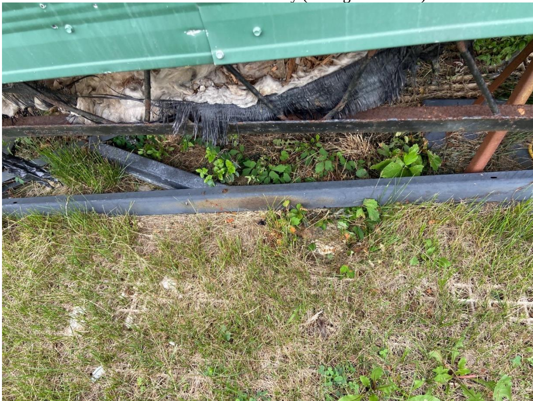
Photo 8: Flush Truck Facility (Facing North)
