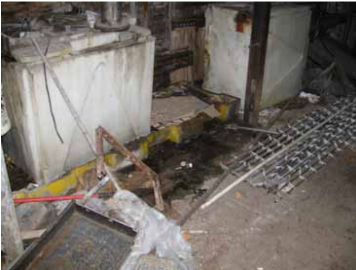
Overflowing chemical storage tanks on an overflowing spill containment pallet. Note the staining in front of the pallet.
