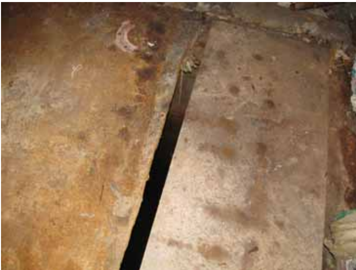
Steel road plates over sump.
