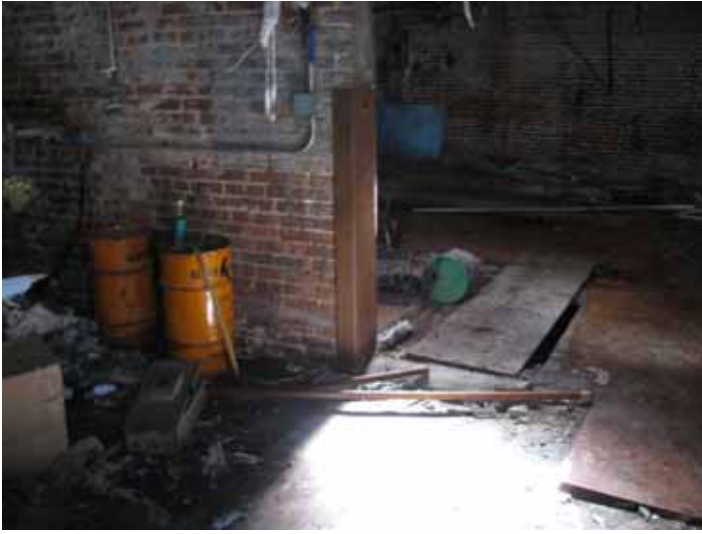
View of grease drums (left) and road plates at the entrance to the southern portion. The gap in the road plates is the location of a sump pit which is full of water.
