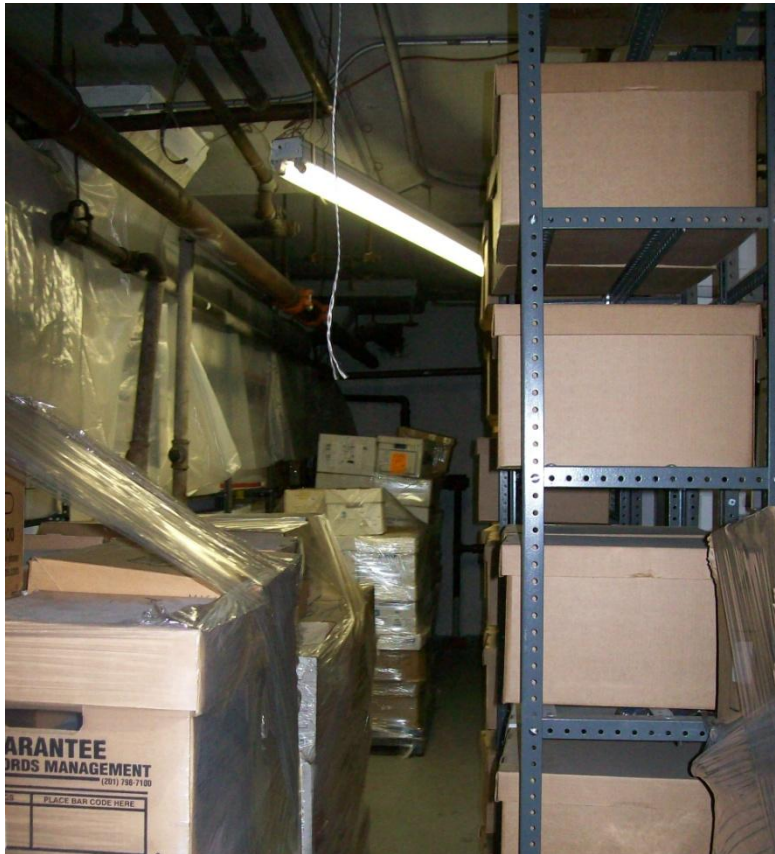
PHOTO 16: Northward view of northern-most portion of CESCO basement.
