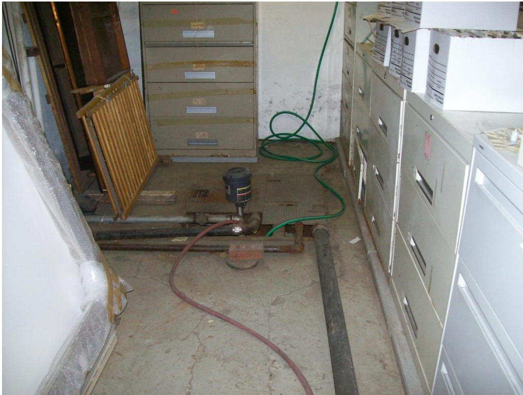
PHOTO 29: Westward view of sump in Bark Frameworks basement.
