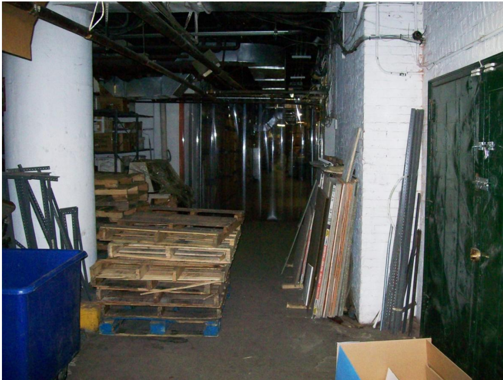
PHOTO 13: Northward view of CESCO basement from door to boiler room.
