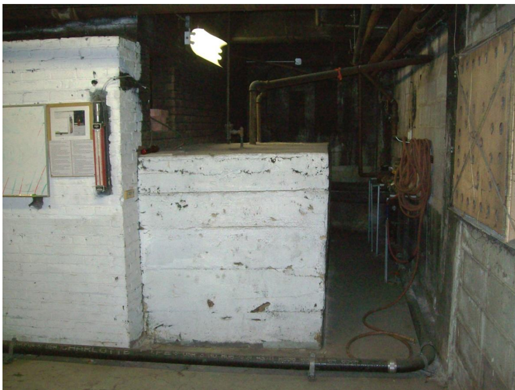
PHOTO 28: Westward view of 1,000 gallon fuel oil tank in Bark Frameworks basement from the bottom of the stairwell.
