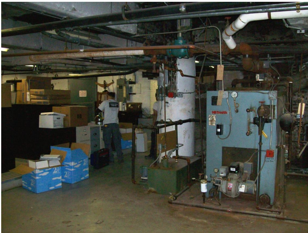
PHOTO 27: Northward view of Bark Frameworks basement.
