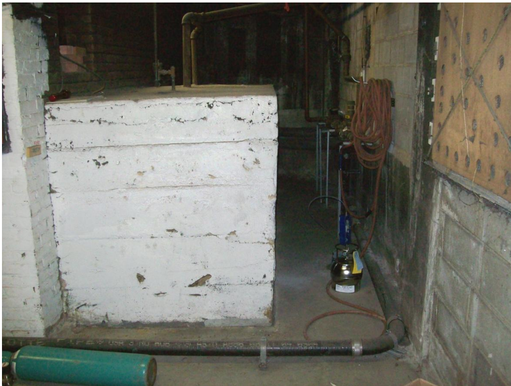
PHOTO 33: Westward view of sub-slab sample BF-SS-2 in Bark Frameworks basement.
