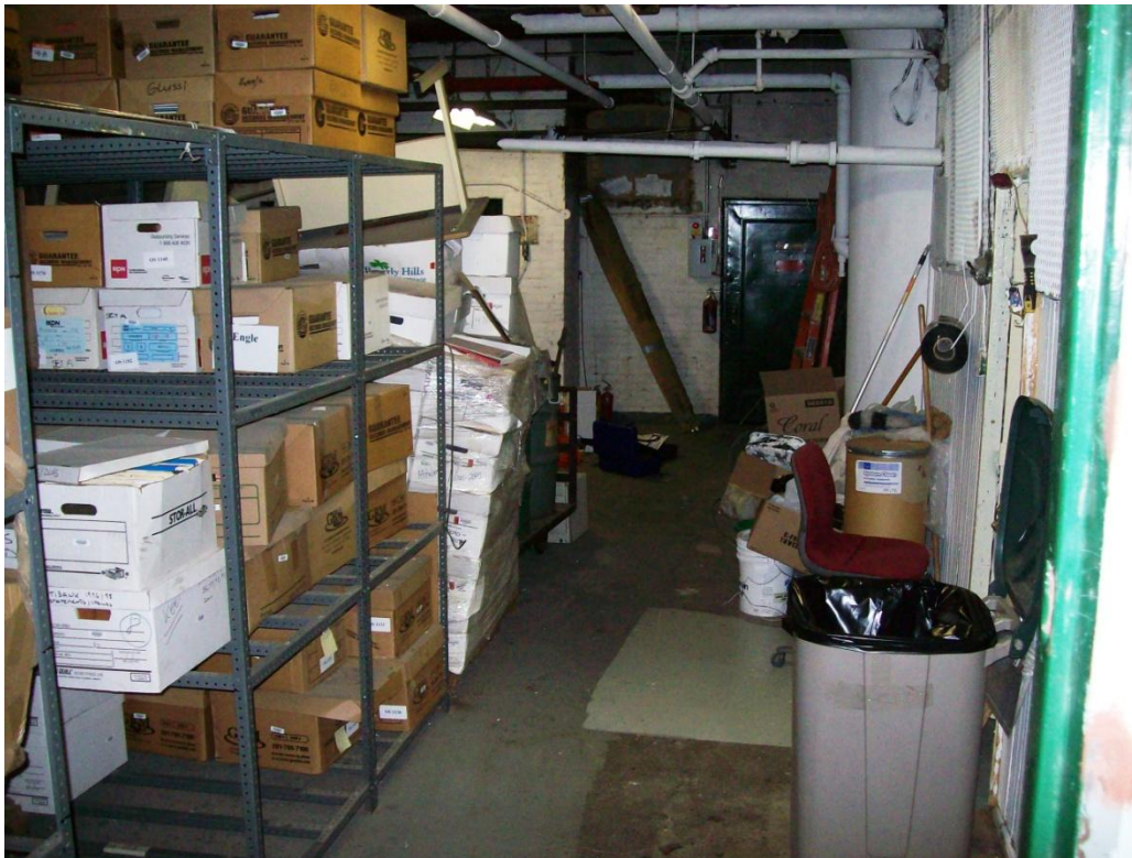
PHOTO 8: Eastward view of CESCO basement. Maintenance office and fuel oil tank to the right, door to boiler room straight ahead.
