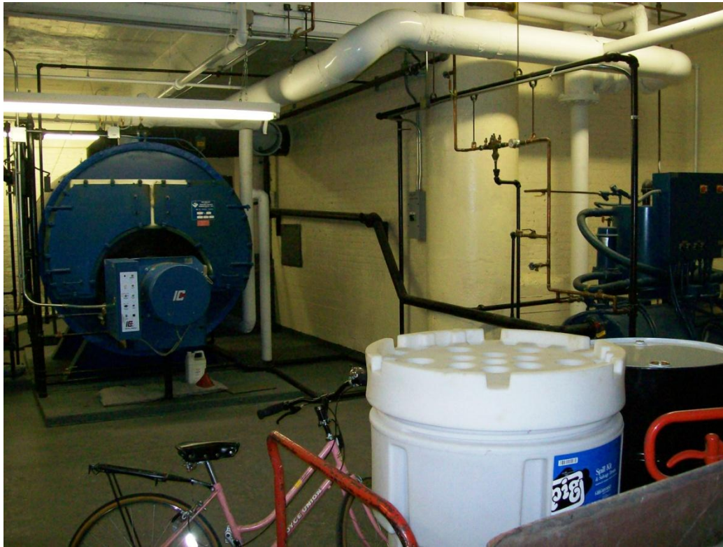
PHOTO 17: Southward view of boiler room in CESCO Basement.
