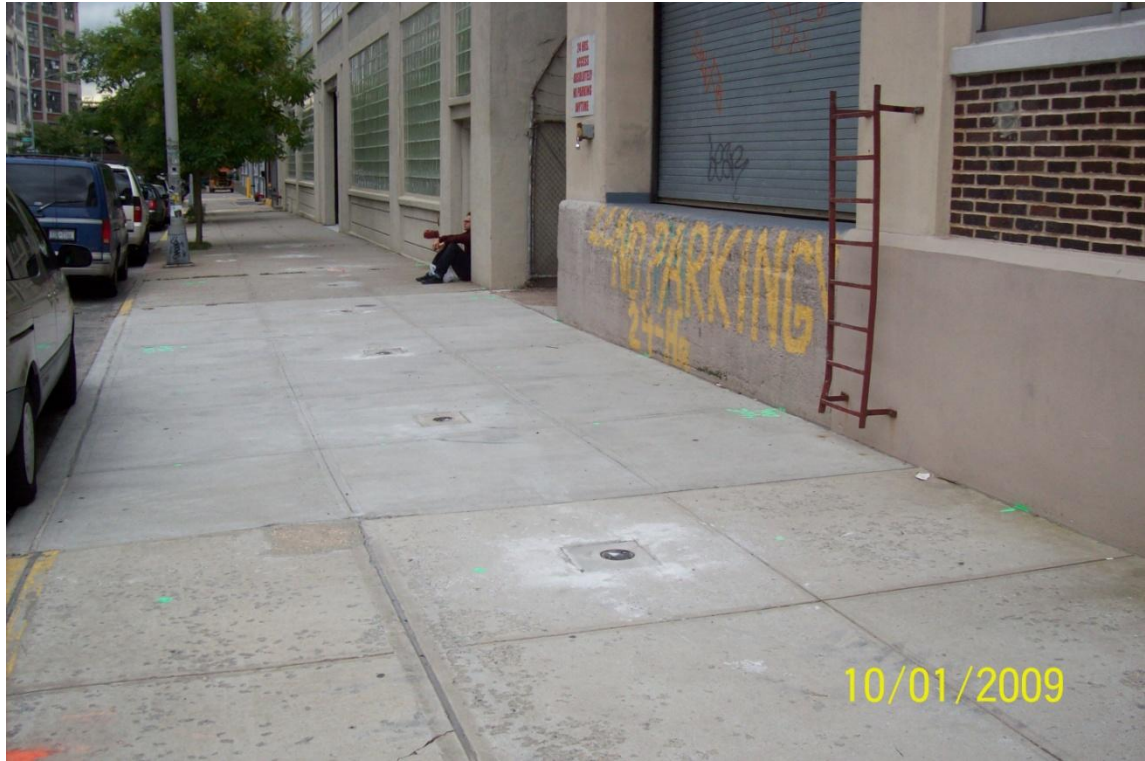
PHOTO 3: Southeast view of 44 th Avenue south sidewalk and extraction points .
