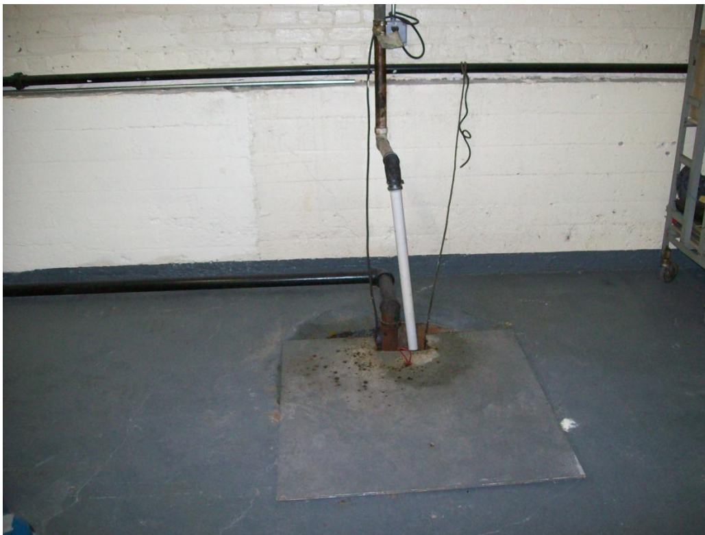
PHOTO 18: Westward view of sump in CESCO boiler room.
