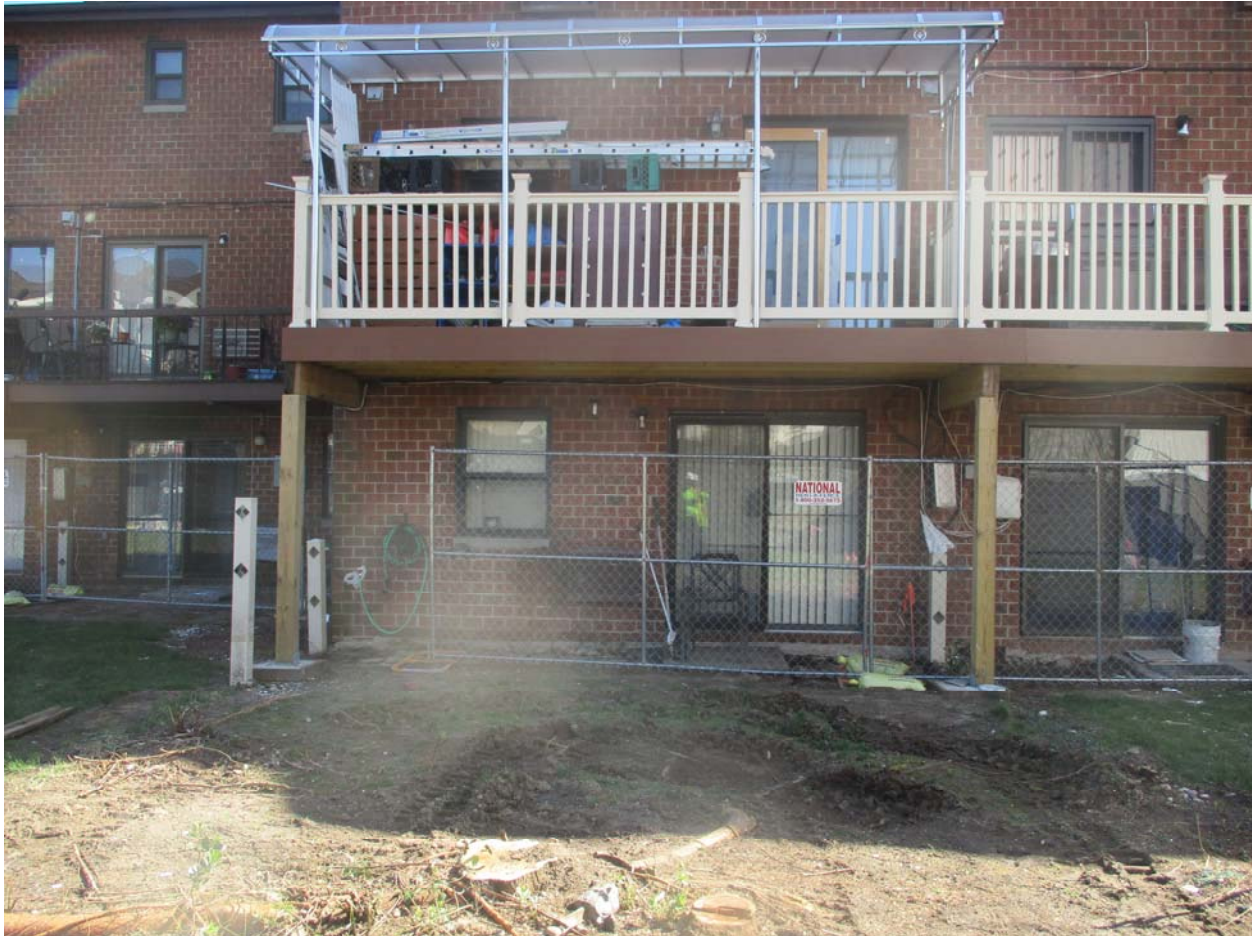
Yard 21: Bricks from Yard 6 shall be used as necessary to restore the patio in this Yard after the completion of excavation and backfill.
