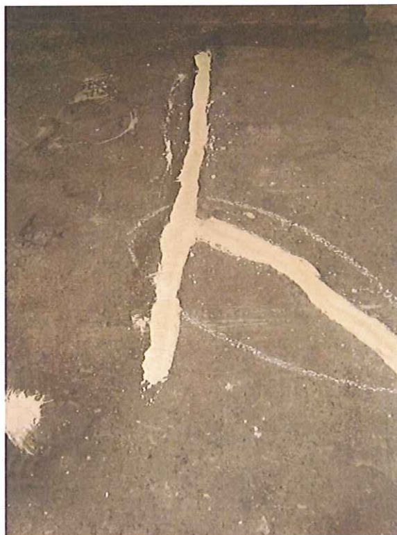
Sealed cracks in floor
