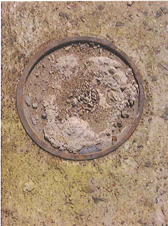
Remote fill port to gasoline UST filled with concrete
