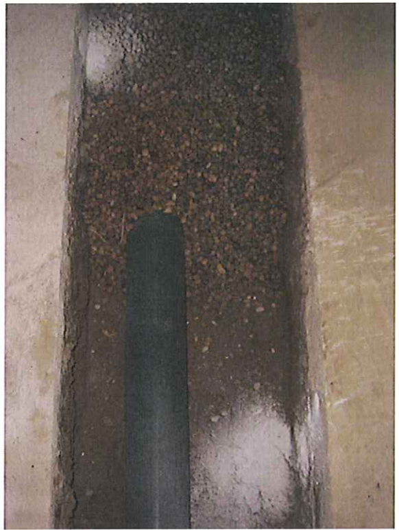
One-half inch diameter gravel placed over pipe in trench
