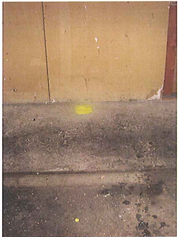
Direct fill port to gasoline UST (marked in yellow) filled with concrete
