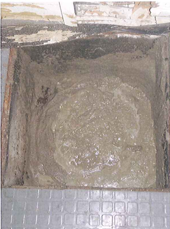
Heating oil UST filled with concrete
