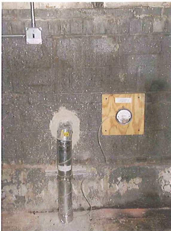
Interior riser pipe with magnehelic guage
