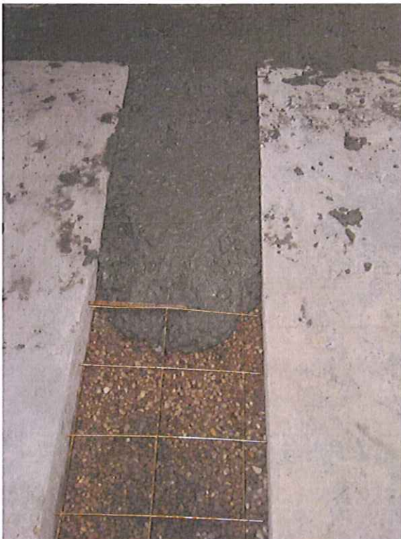
Concrete placed over pipe and gravel in trench
