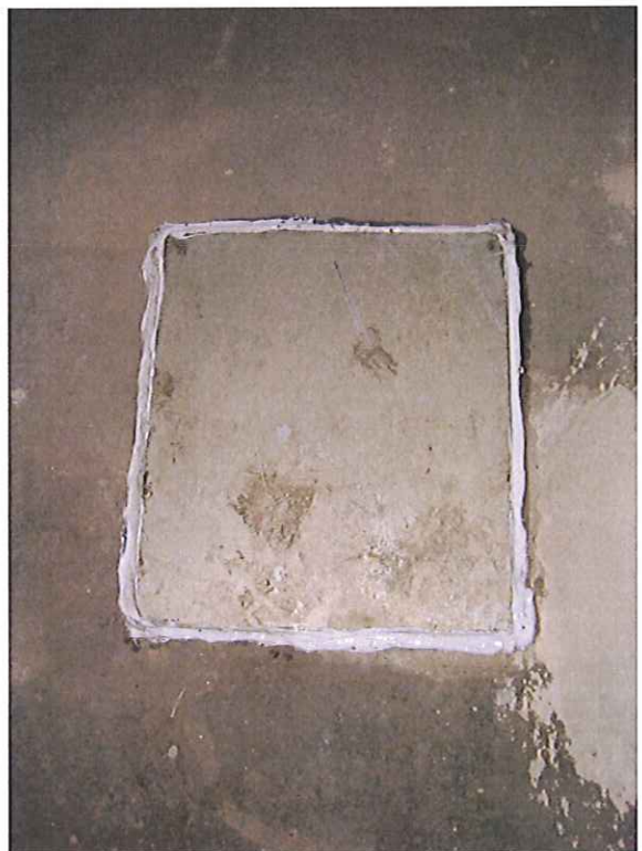
Metal cover sealed over floor pit
