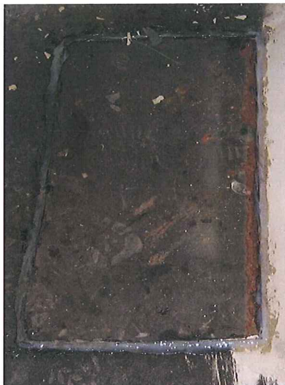
Metal cover sealed over floor pit
