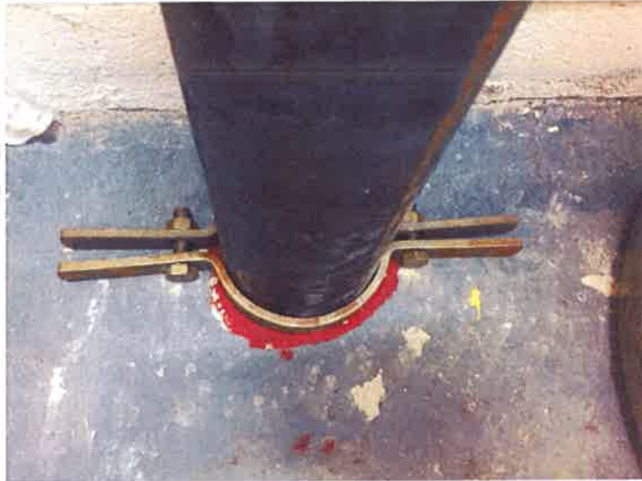
Photo 4 (October 12, 2018): Floor penetration has been firestopped.
