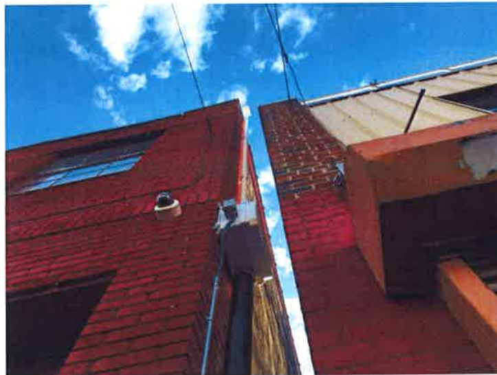
Photo 3 (October 12, 2018): View of installed exhaust stack and fan.
