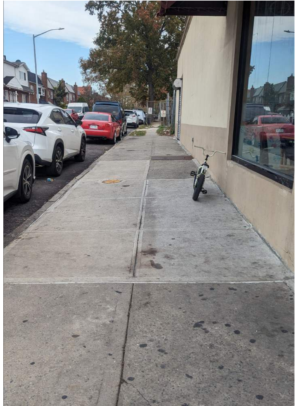
Sidewalk along Selover Road (NW of building)
