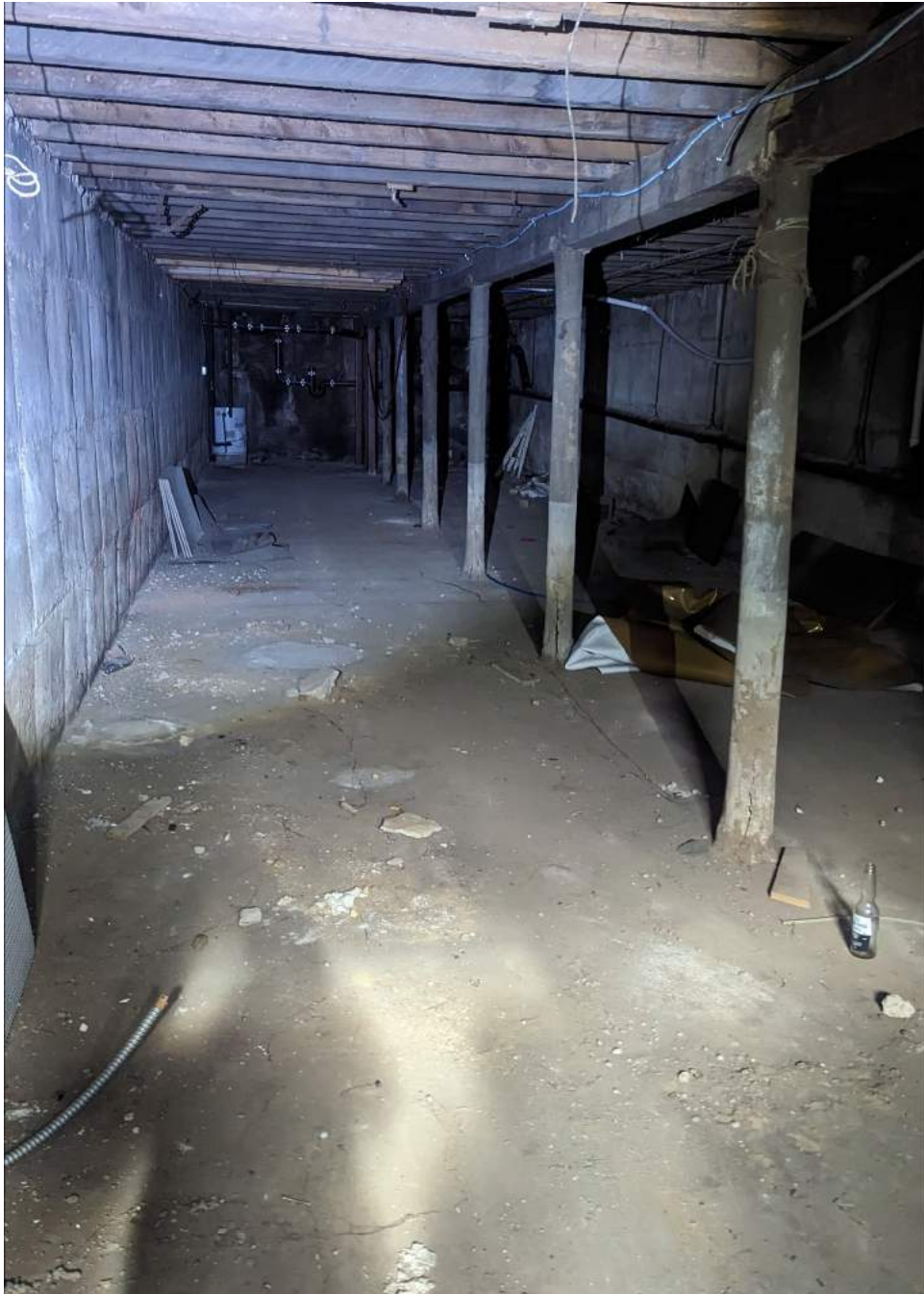
BASEMENT OF UNIT 127-09
