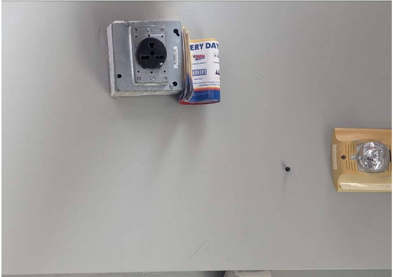
SSDS WARNING LIGHT AND ALARM IN UNIT 127-03
