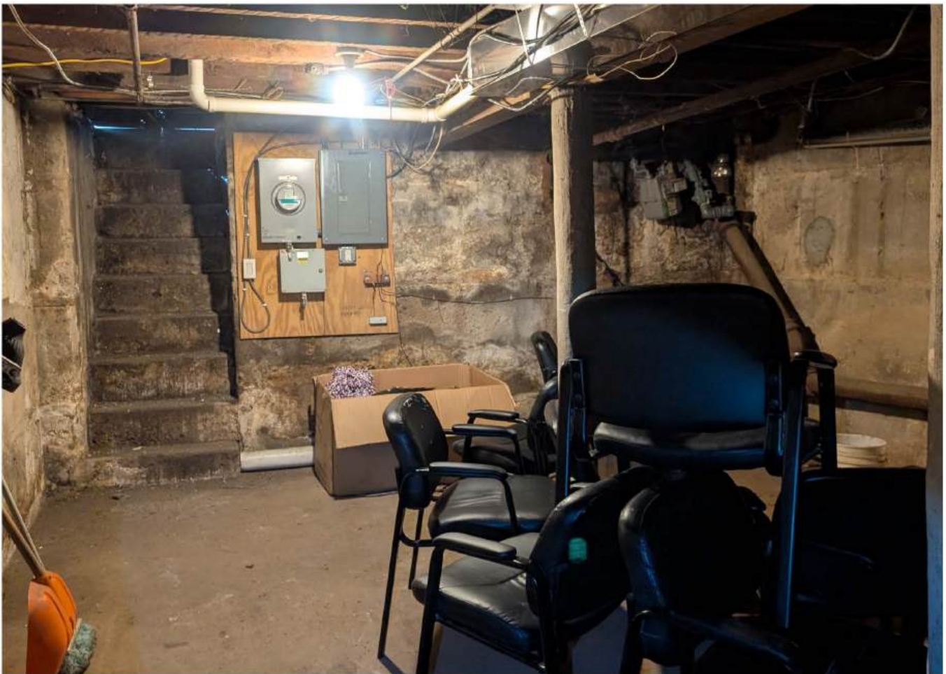
BASEMENT OF UNIT 127-11
