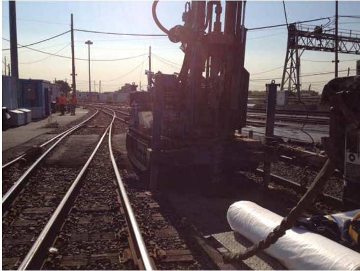
Photograph 9. Advancing soil boring at MW-39S.
