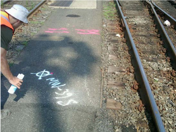
Photograph 1. Geophysical markout of MW-39S
