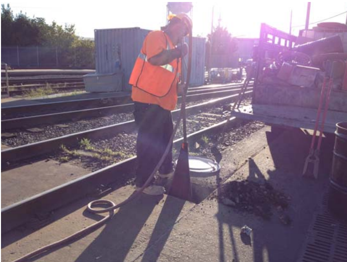
Photograph 3. Hand clearing at second attempt location for MW-38S.
