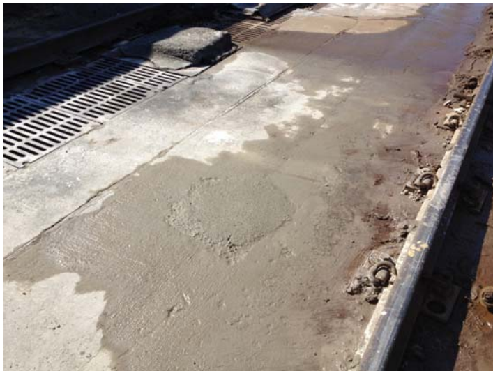
Photograph 11. Concrete repair at MW-38S.
