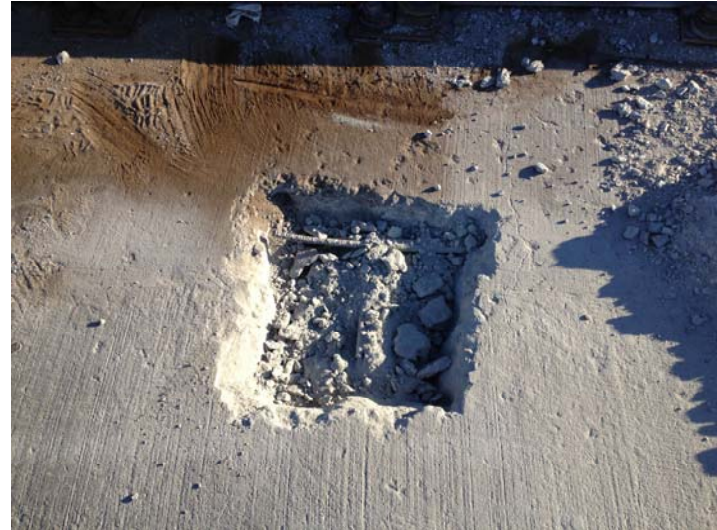
Photograph 2. Concrete removal at MW-38S, note presence of rebar.
