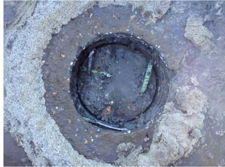
Photograph 10. Rebar in 10-inch coring at MW-38S.
