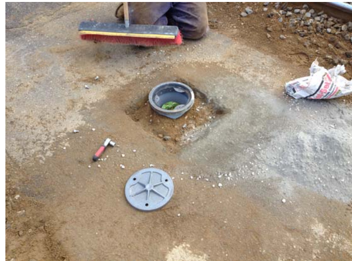
Photograph 12. Monitoring well installation at MW-39S.
