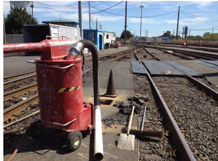
Photograph 8. Hand clearing at MW-39S.
