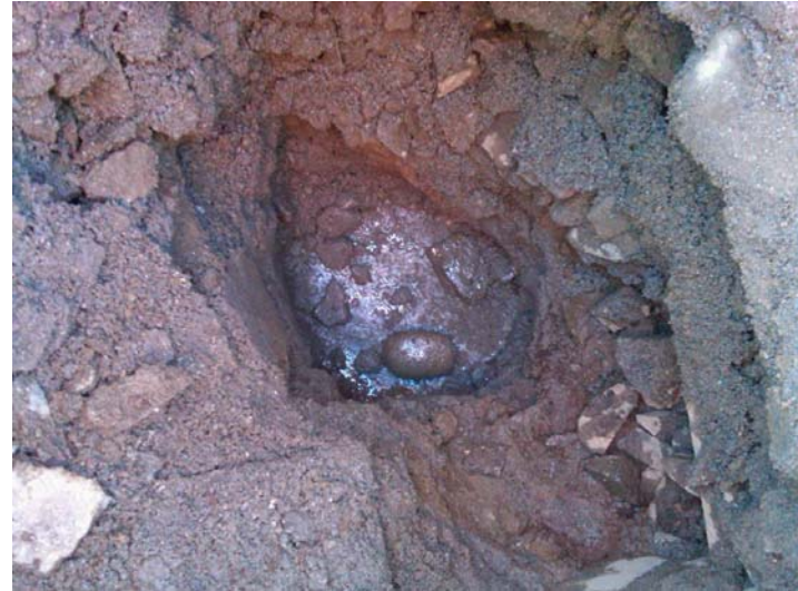
Photograph 6. Subsurface structure encountered at approximately 2 feet below ground surface at third attempt location for MW-38S.
