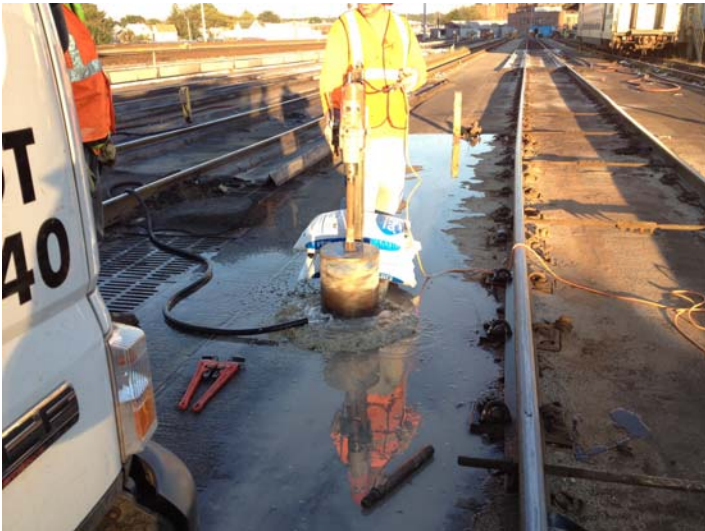
Photograph 7. Coring at original location of MW-38S.
