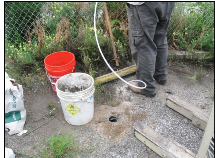
Photograph 4: Soil vapor point installation at SV-9.
