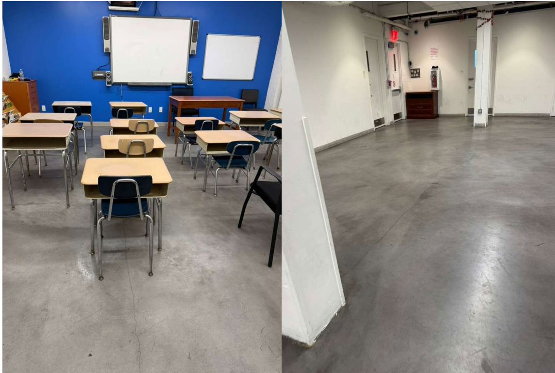
View of fine cracks in the basement slab
