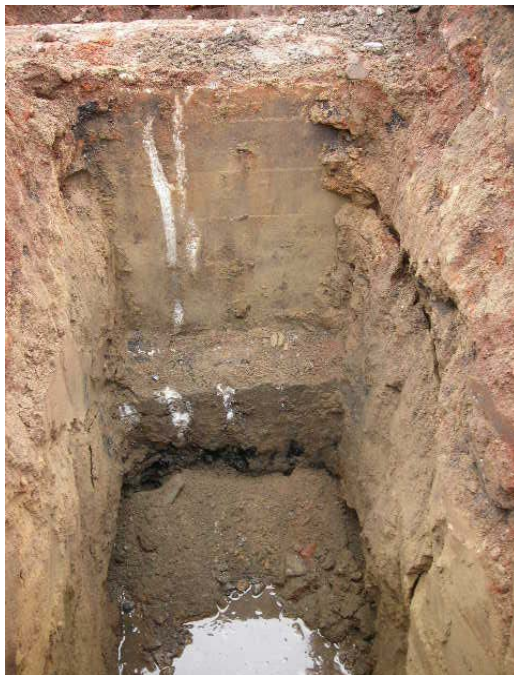
Excavation closeup From the West
