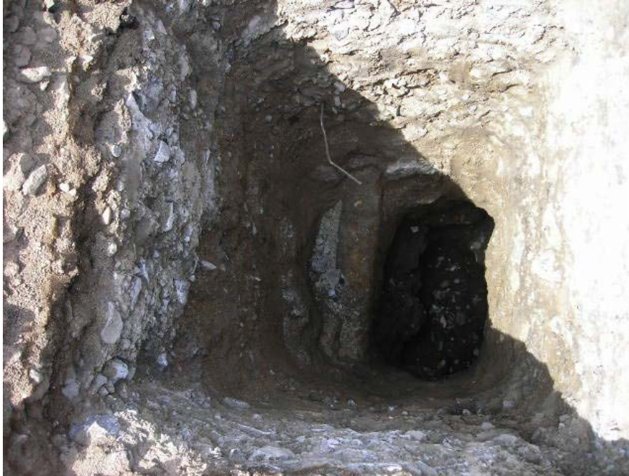
Above: Metal rail/rod encountered at approximately 3 ft bgs
