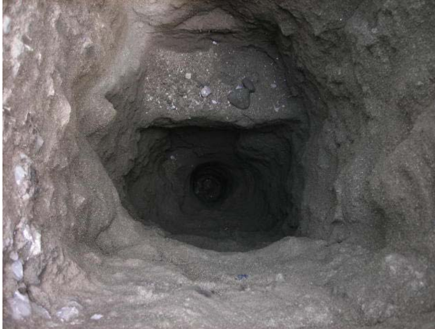
Above: Edge of holder encountered at 4 ft bgs on east side of hand clearance hole.
