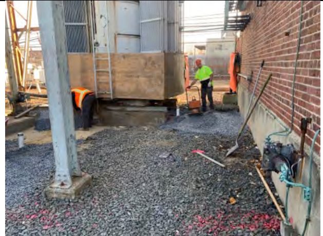
Aarco compacting stone.
