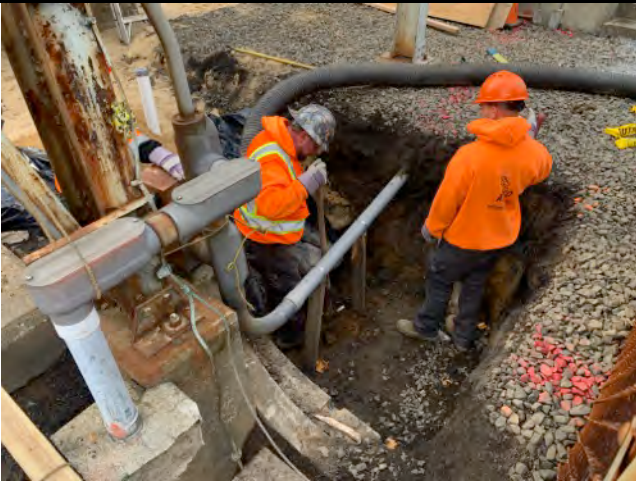
Aarco continues to backfill the western portion of area #3.
