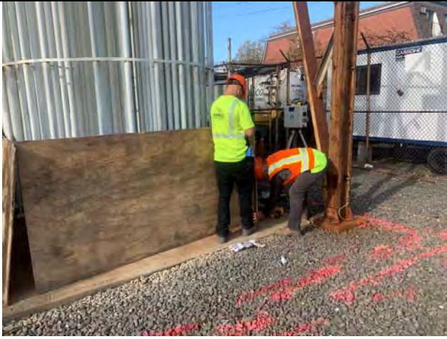
Protecting transformers.
