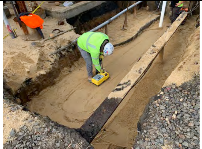
Soil Mechanics performing compaction testing.
