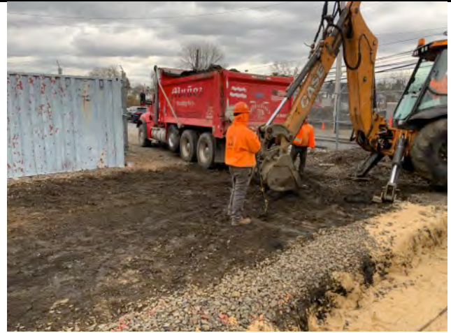
Scrapping the former stockpile area to ensure all soils are transported offsite.
