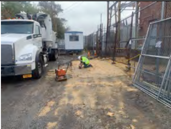
Soil Mechanics conducting compaction testing.
