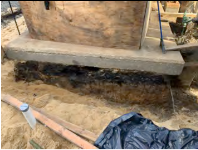
Aarco continues to excavate the along the western side of the transformer slab.
