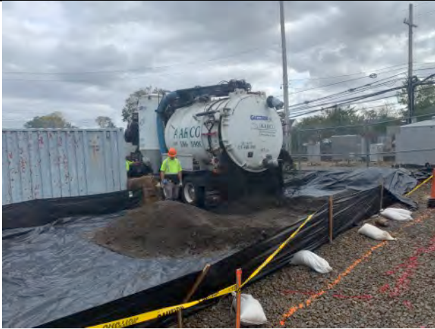
Dumping soils excavated from area #2 within stockpile area.
