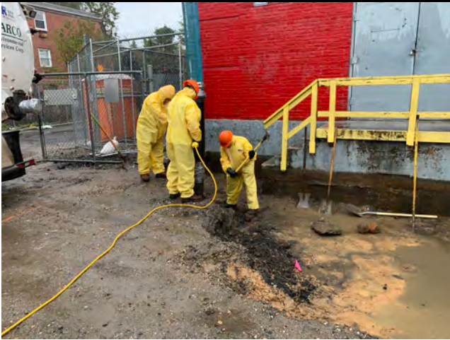
Continuing to excavate soils from area #2.
