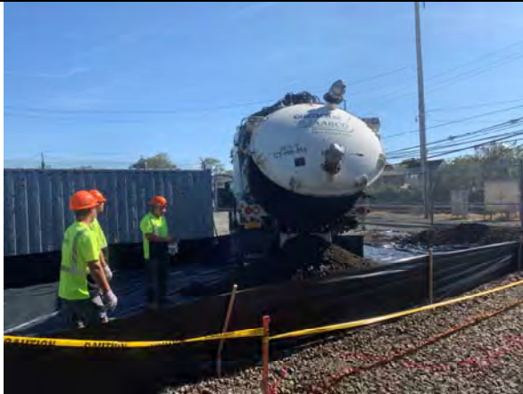
Dumping soils excavated from area #2 within new stockpile area.
