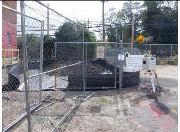
Stockpile area for all soils excavated from Area #1.
