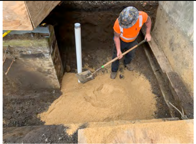
Aarco installing PVC tube to allow survey of endpoint samples.
