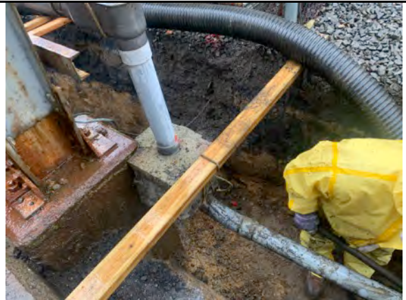
Continue excavation of Area #3.
