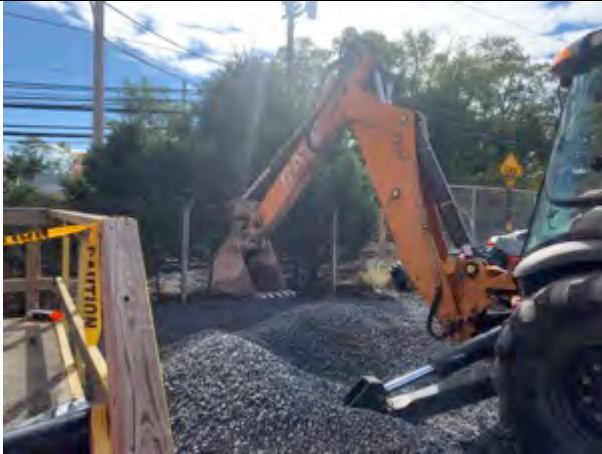
Spreading stone in area #2.
