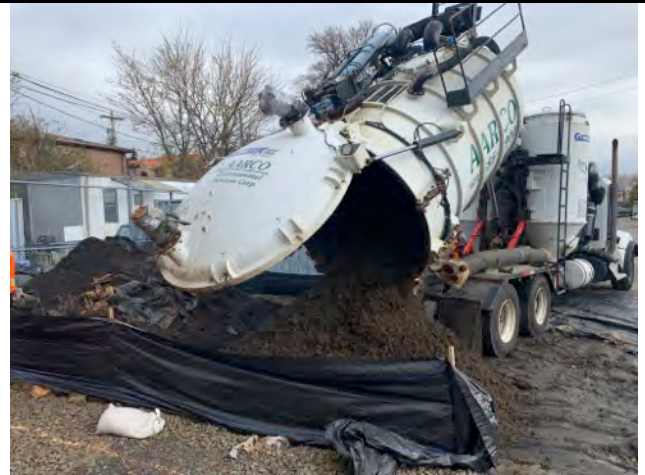
Aarco dumping soils onto the stockpile from the guzzler truck.
