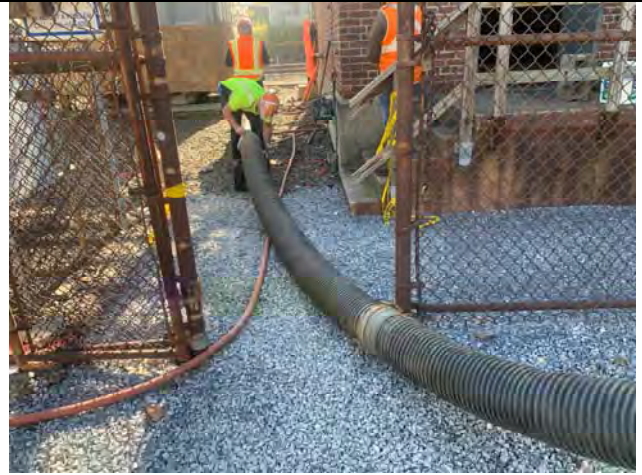
Utilizing guzzler truck to remove soils from area #3.
