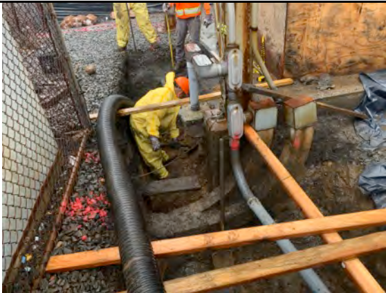
Excavating on the north side of the transformer pad.
