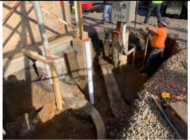
Aarco installing PVC tube to allow endpoint samples to be surveyed.
