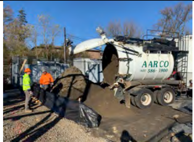
Aarco dumping guzzler truck onto stockpile.
