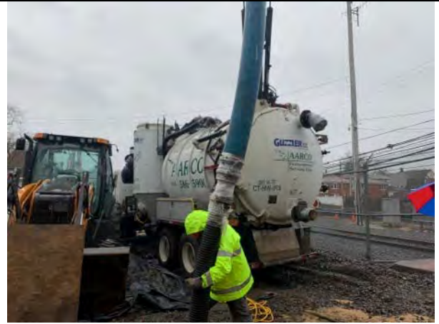
Aarco utilized guzzler truck to remove all soils.
