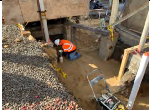
Soil Mechanics testing backfill for 95% compaction, all lifts pass.
