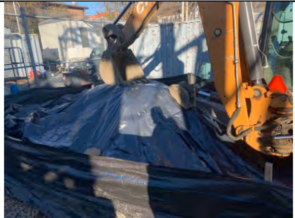
Aarco covering stockpile at the end of the day.
