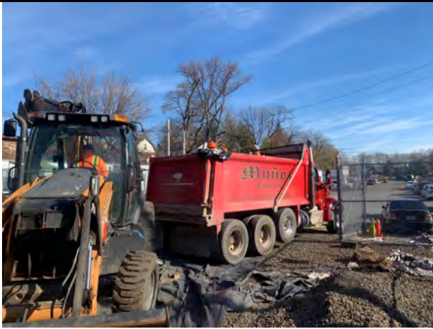
Aarco installing liner to truck prior to loading soils for disposal.
