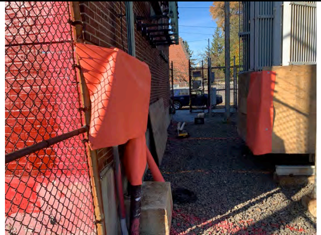
Wrapping junction box in protective material for duration of excavation.
