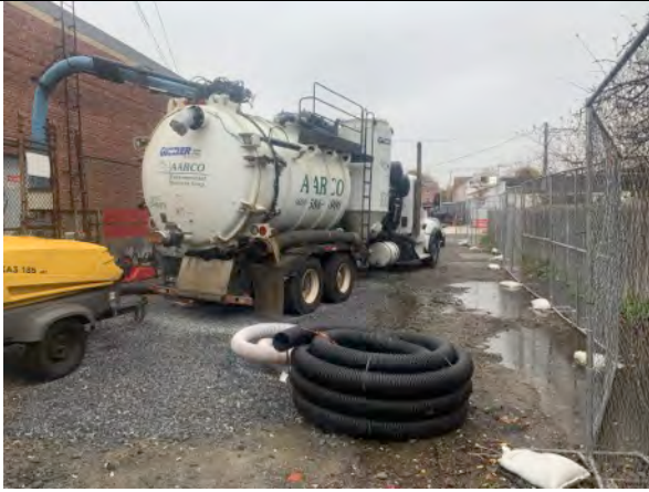
Utilizing guzzler truck to continue to remove soils from area #3.
