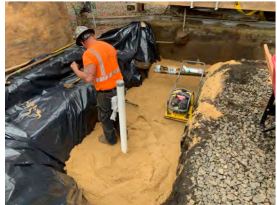
Aarco compacting backfill in ten (10) inch lifts with compactor.
