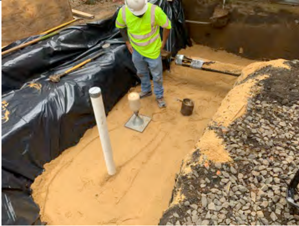
Soil Mechanics onsite to preform compaction testing.
