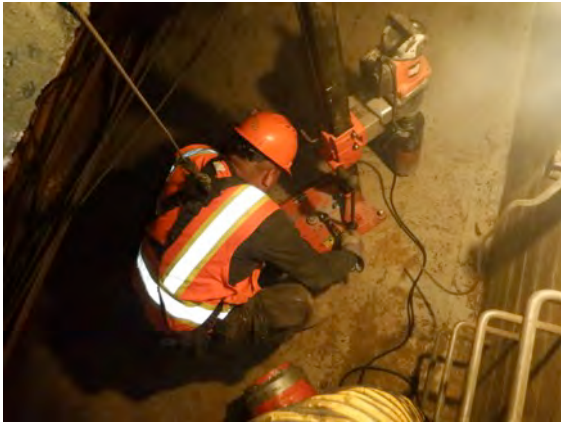
Aarco core drilling substation slab to collect BSBEP-2.
