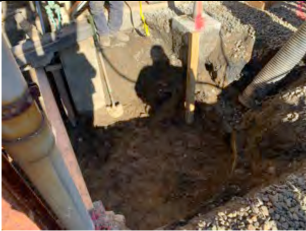
Aarco installing wooden supports to all exposed conduits.
