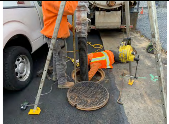
Aarco cleaning out soils from area #4.
