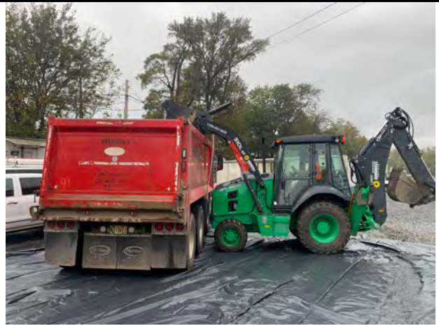
Loading out soils for transport and disposal at Clean Earth.
