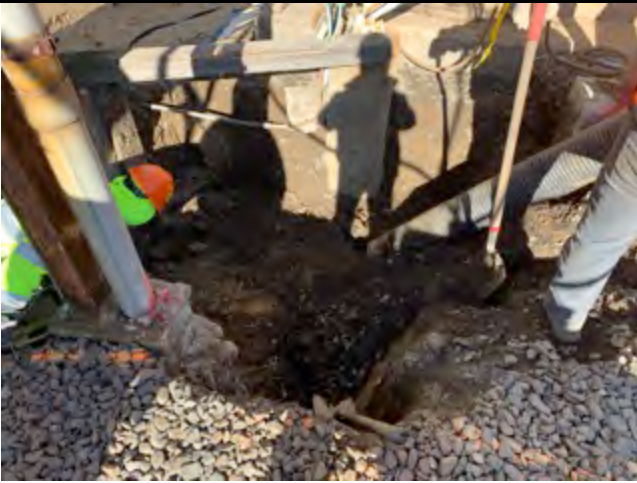
Aarco continues to excavate the souther side of Area #3.
