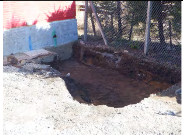
Area #2 excavated at the end of the day.
