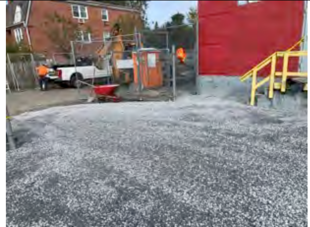
Backfill completed in Area #2 .
