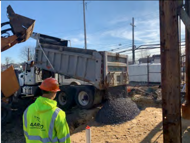
Aarco backfilling with 3/4 inch stone.
