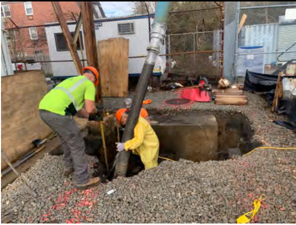
Aarco continues excavating area #3.
