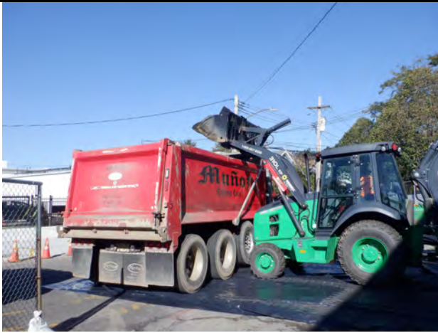
Loading out soils from Area #1.
