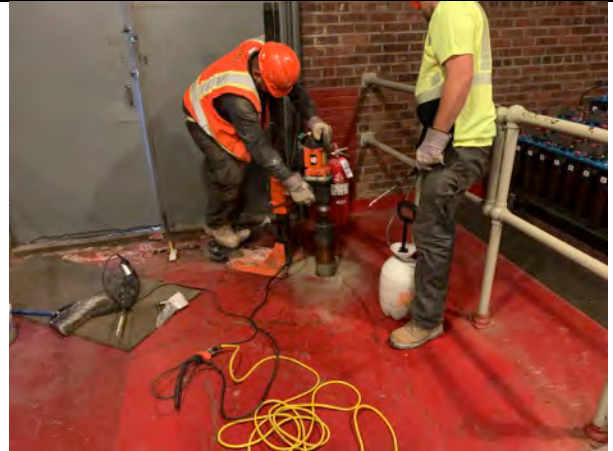
Aarco core drilling BSBEP-3.
