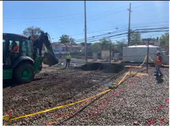
Aarco clearing new stockpile area outside of area #3.
