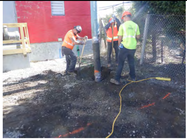
Starting excavation of area #2.
