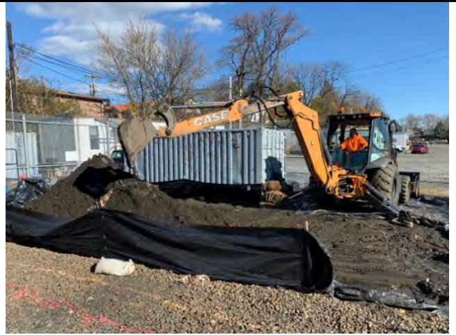
Aarco moving soils onto stockpile to make room.
