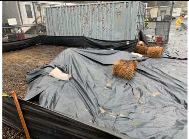
Securing the stockpile at the end of the day.
