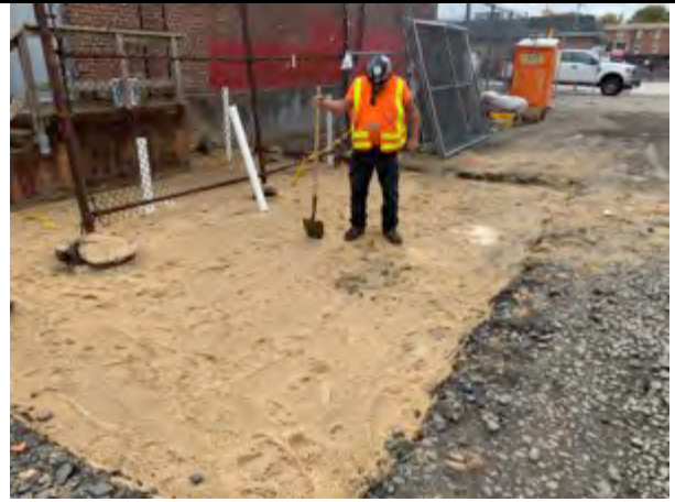
Backfilling and compacting endpoint sample markers.
