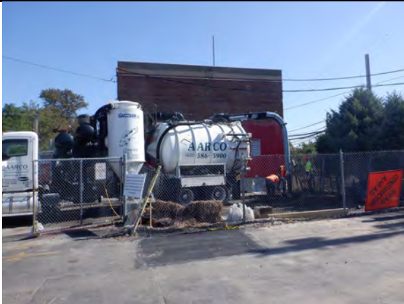
Area #2 excavated via a soil guzzler.
