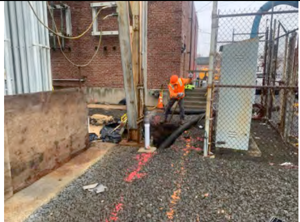
Continue excavation of Area #3.
