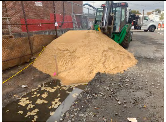
Starting to backfill area #1.
