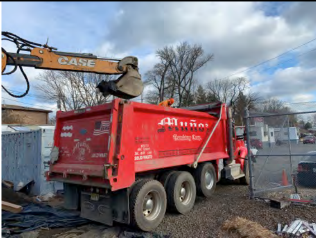
Loading out soils for disposal.
