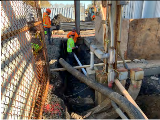
Aarco continues excavating within area #3.
