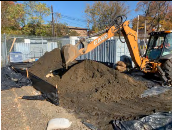
Moving stockpiled soils.
