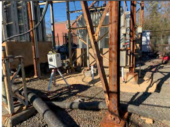
Work zone camp monitoring station.
