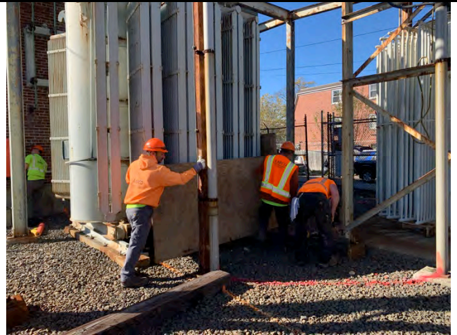
Aarco installing plywood protections.
