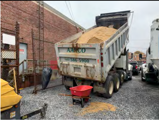
Sand utilized to backfill area #3.
