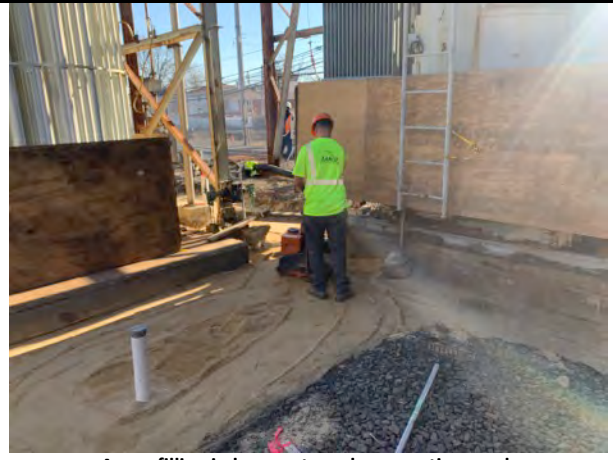
Aarco filling in low spots and compacting sand.
