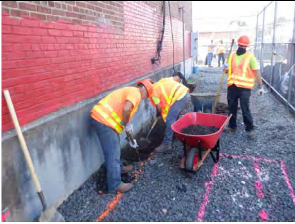
Excavating soils from area #1.
