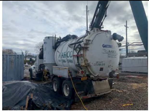
Aarco utilizing the guzzler truck to excavate all soils.
