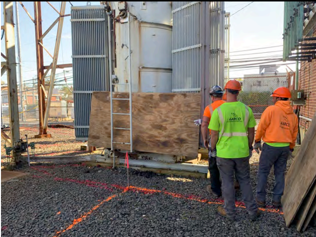
Aarco installing plywood protection around transformer.
