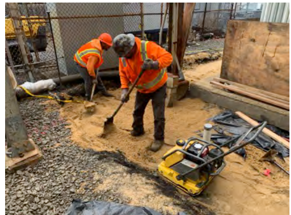
Aarco utilizing a gas compactor when conduit was backfilled.
