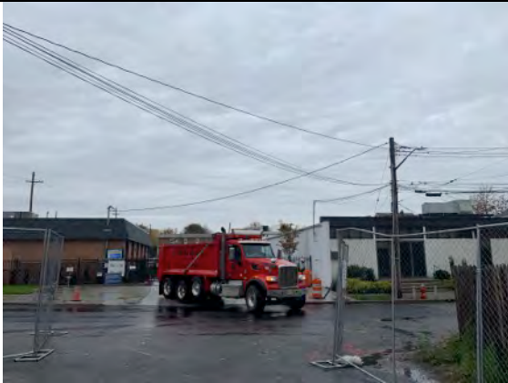
Aarco loading out two trucks for transport to Clean Earth.
