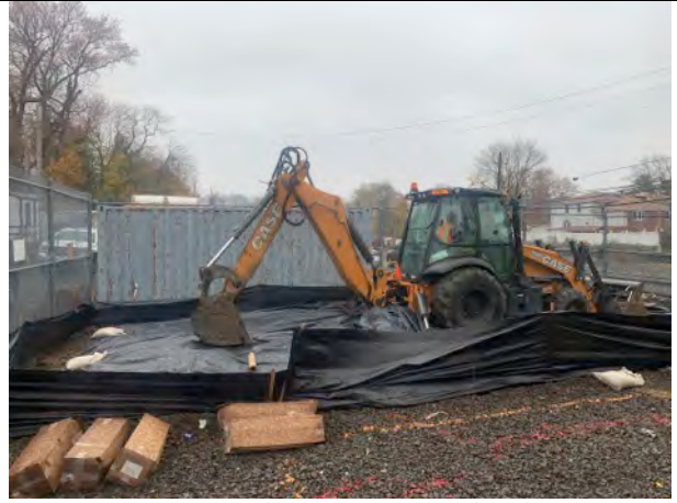
Laying down new plastic in stockpiling area.
