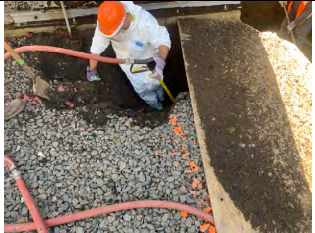
Utilizing guzzler truck and air knife to remove soils from area #3.
