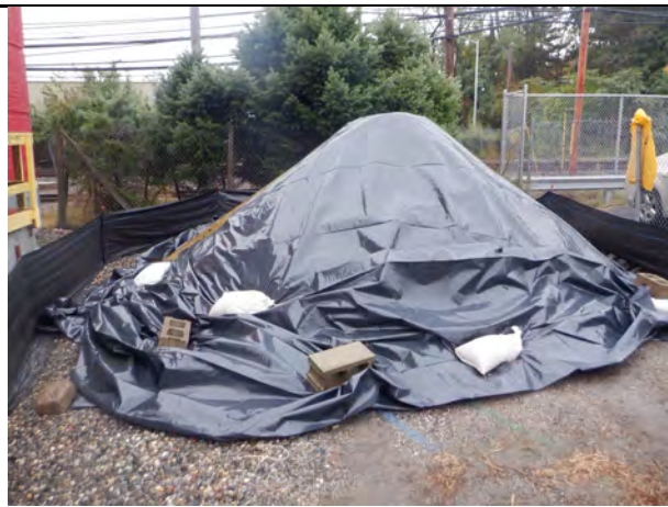
Securing the stockpile at the end of the day.
