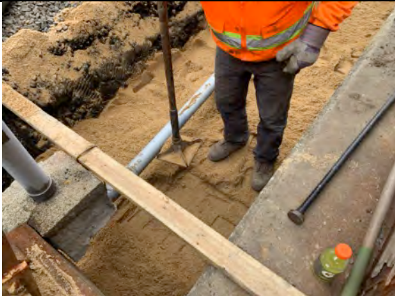
Aarco utilizing a hand tamper around conduits to compact backfill.
