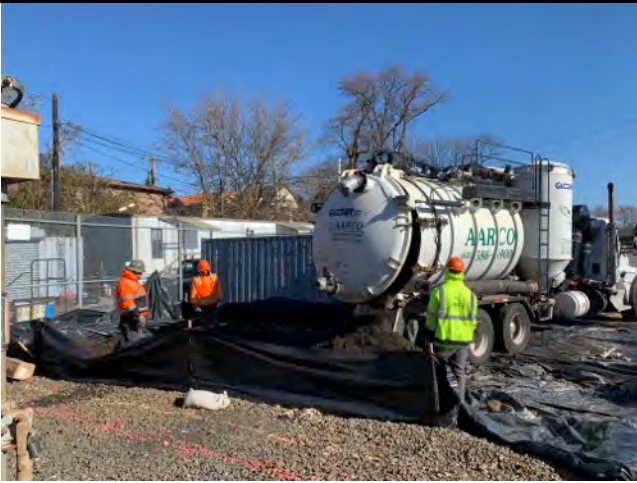
Aarco dumping guzzler truck onto stockpile.
