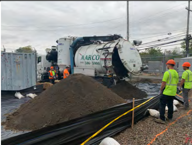
Dumping soils excavated from area #2 on to stockpile.
