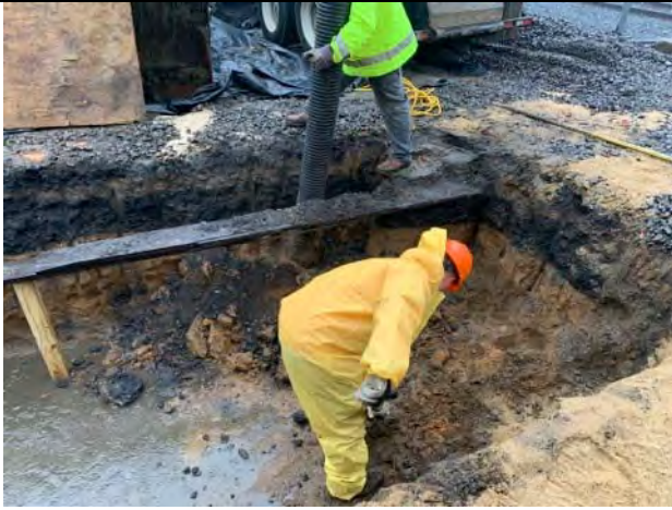
Aarco removing soils from the southern portion of area #3.
