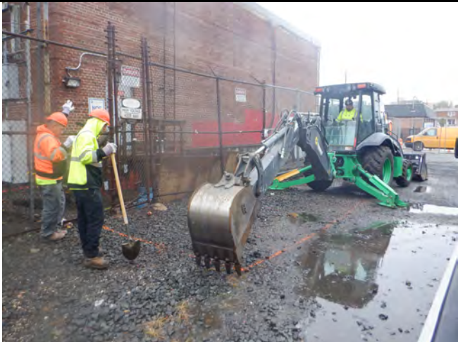
Continuing to excavate soils from area #1.
