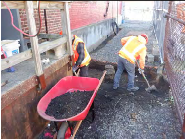
Continuing to excavate soils from area #1.
