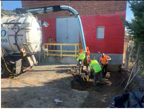
Continue excavating from area #2.
