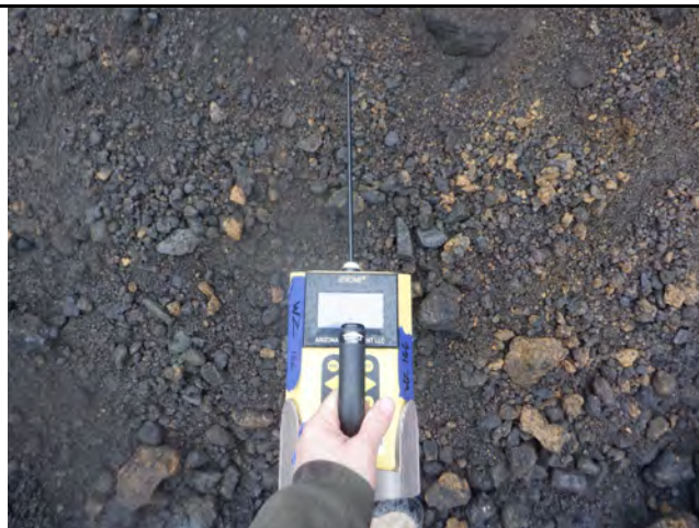
Screening soils for mercury during excavation of area #1
