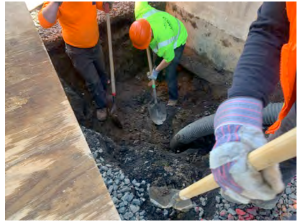
View of excavation in area #3.
