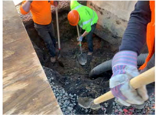
View of excavation in area #3.
