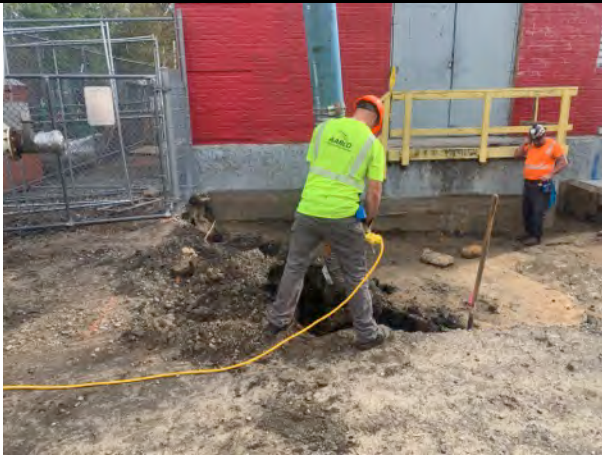
Continue excavating from area #2.
