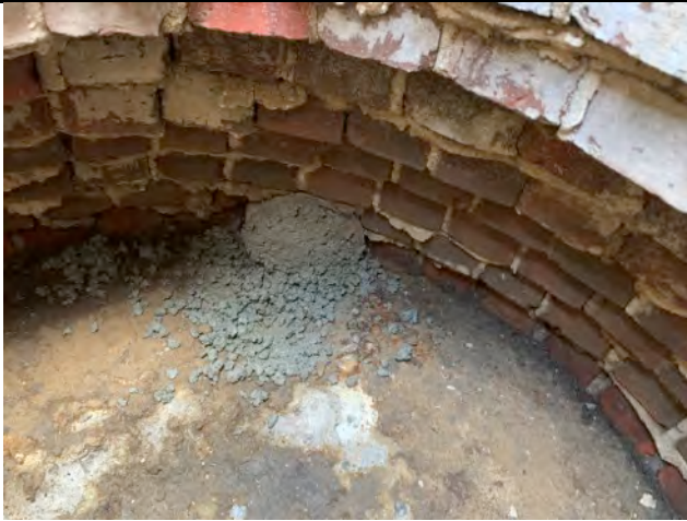
Bulk heading storm sewer pipe in area #4.
