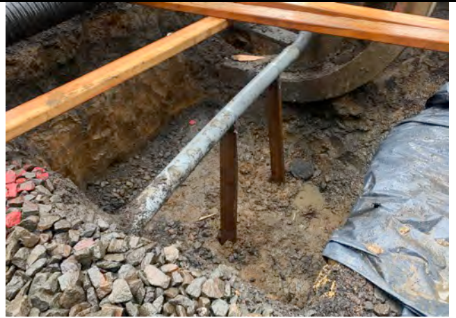
Supporting uncovered conduit during excavation.
