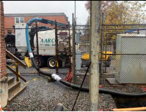
Utilizing guzzler truck to continue to remove soils from area #3.
