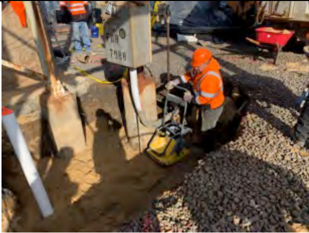
Aarco compacting all backfill with a gas compactor.
