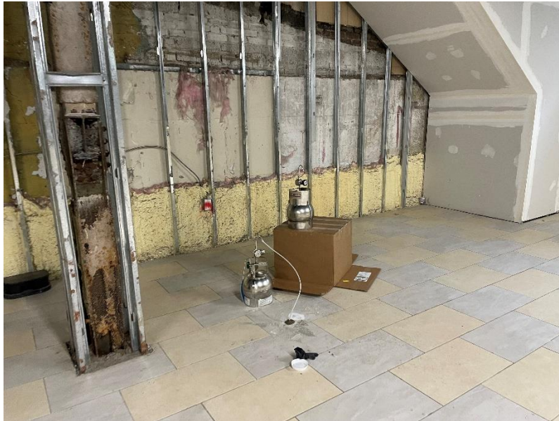
Photo 1: View of soil vapor sampling at HA SS-07, facing Southeast.
