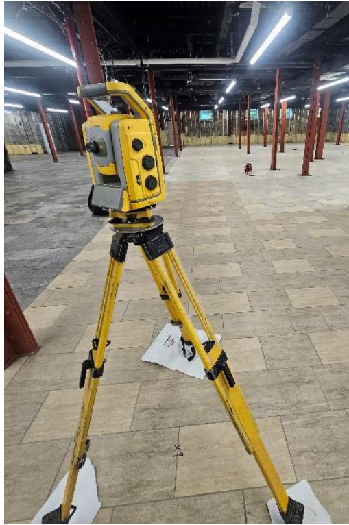
Photo 1: View of contractor surveying monitoring wells, facing east.
