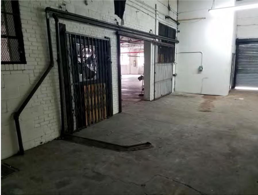
5. Fill and vent lines showing the area of 2,000-gallon fuel oil underground storage tank (UST), located at southern-central portion of warehouse
