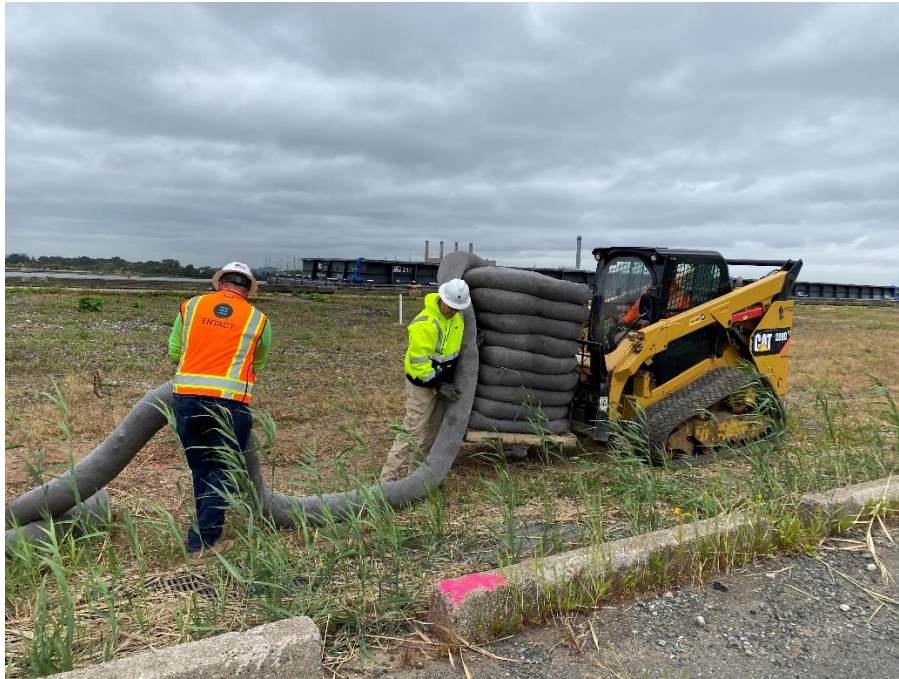
Photo 1: View of Entact installing E&S controls along the trench drain in IRM 1 Eastern Area, facing west.
