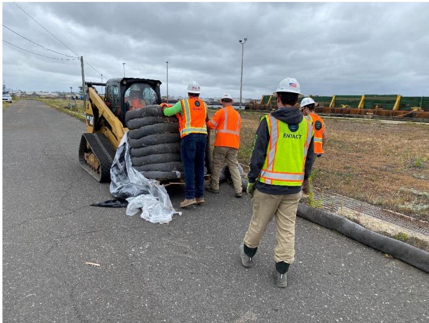
Photo 2: View of Entact installing E&S controls along the trench drain in IRM 1 Central Area, facing south.
