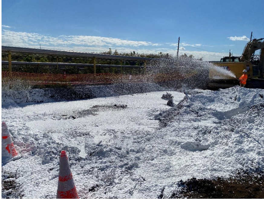
Photo 1: View of Entact spraying Rusmar odor suppression foam in Excavation 5, IRM 1 Eastern Area, facing southeast.
