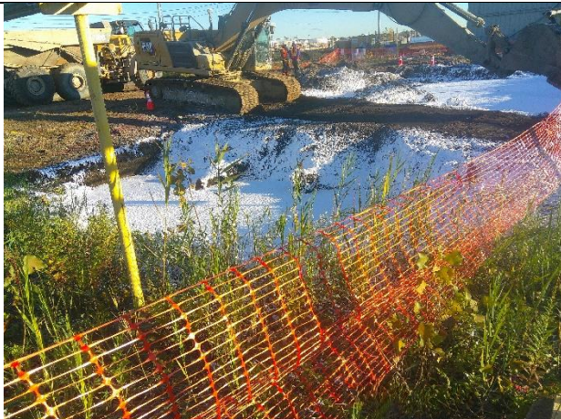
ENTACT sprayed odor-suppression foam at excavation #5.
