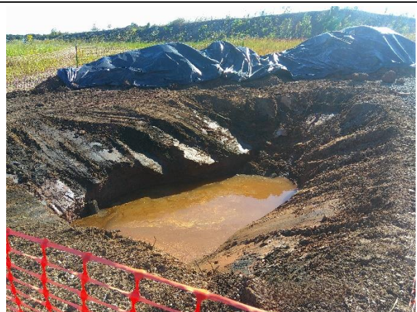
Test pitting at excavation #9 to determine water depth
