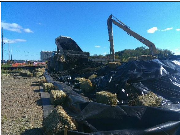
Stockpile containment pad
