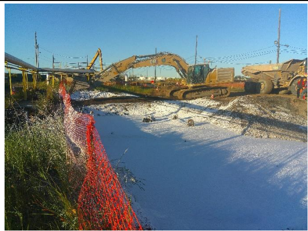
ENTACT sprayed odor-suppression foam at excavation #5 in the morning before excavating.
