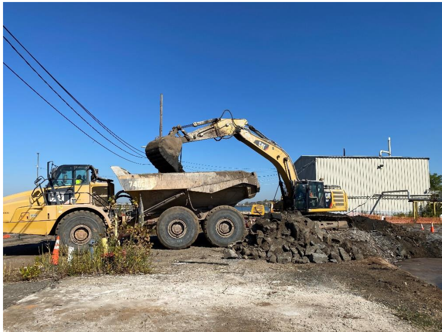
Photo 2: View of soil loading onto rock truck for staging in containment area, in Excavation 5, IRM 1 Eastern Area, facing north.
