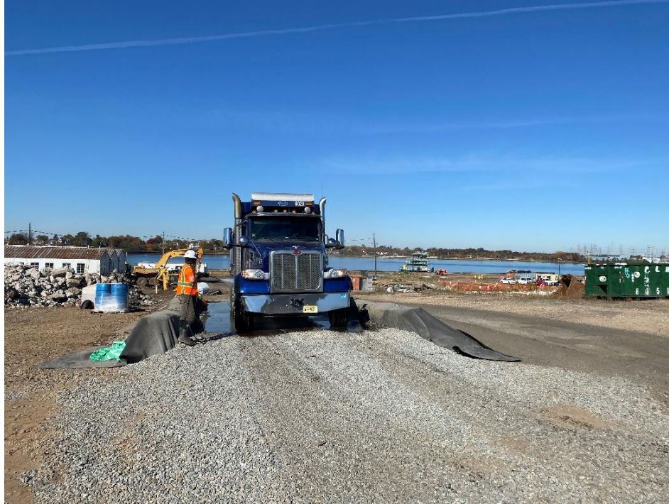
Photo 1: View of truck washing station in IRM 1 Central Area, facing west.
