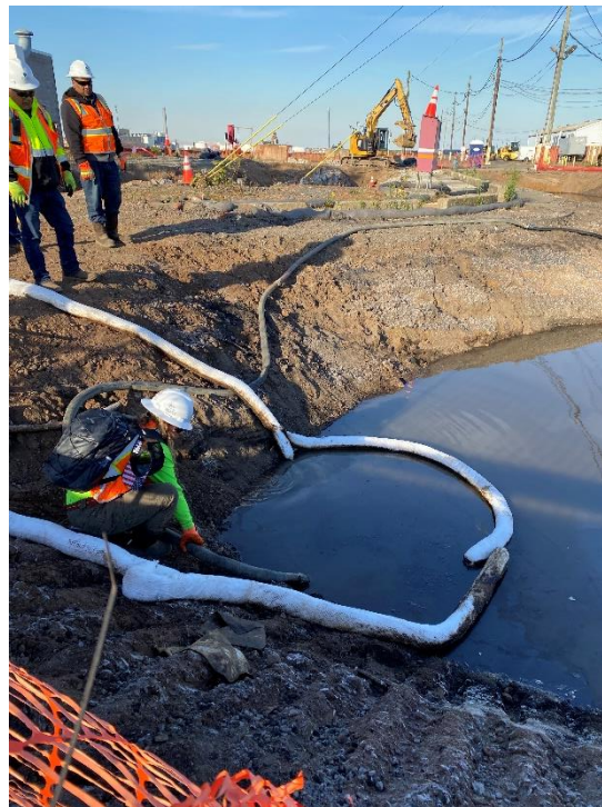
Photo 2: View of LNAPL collection using absorbent sock in Excavation 1, IRM 1 Western Area, facing north.
