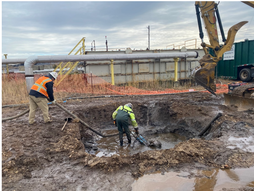
Photo 4: View of Excavation 6B dewatering activities, IRM 1 Eastern Area, facing east.
