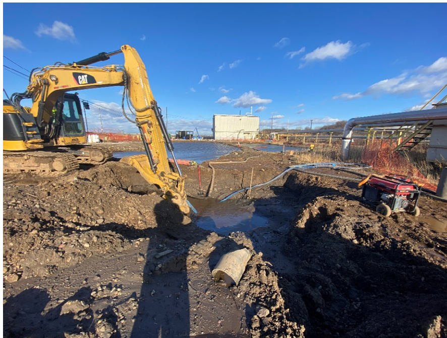
Photo 4: View of Excavation 6B dewatering activities, IRM 1 Eastern Area, facing north
