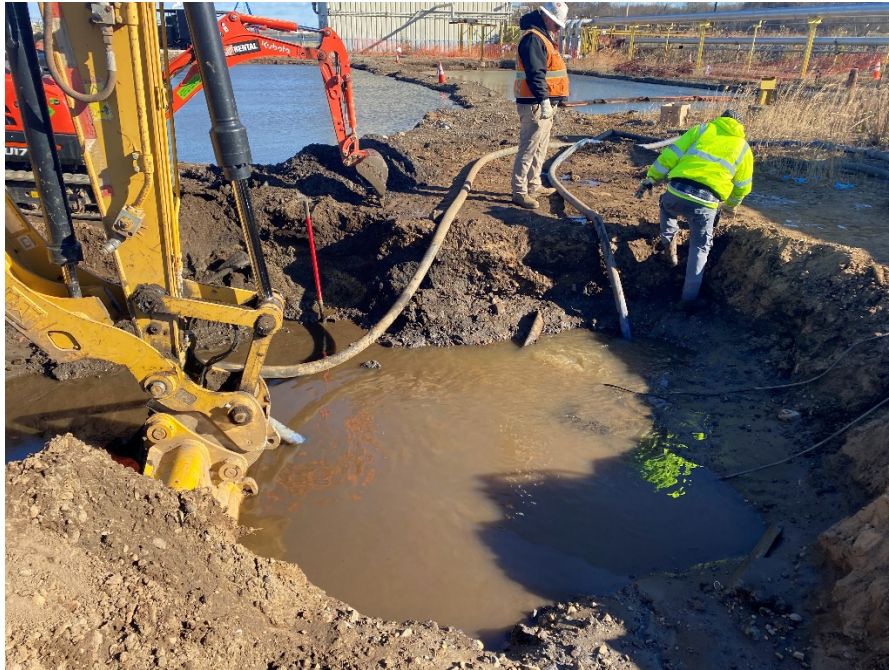
Photo 1: View of dewatering activities in Excavation 6A, IRM 1 Eastern Area, facing south.
