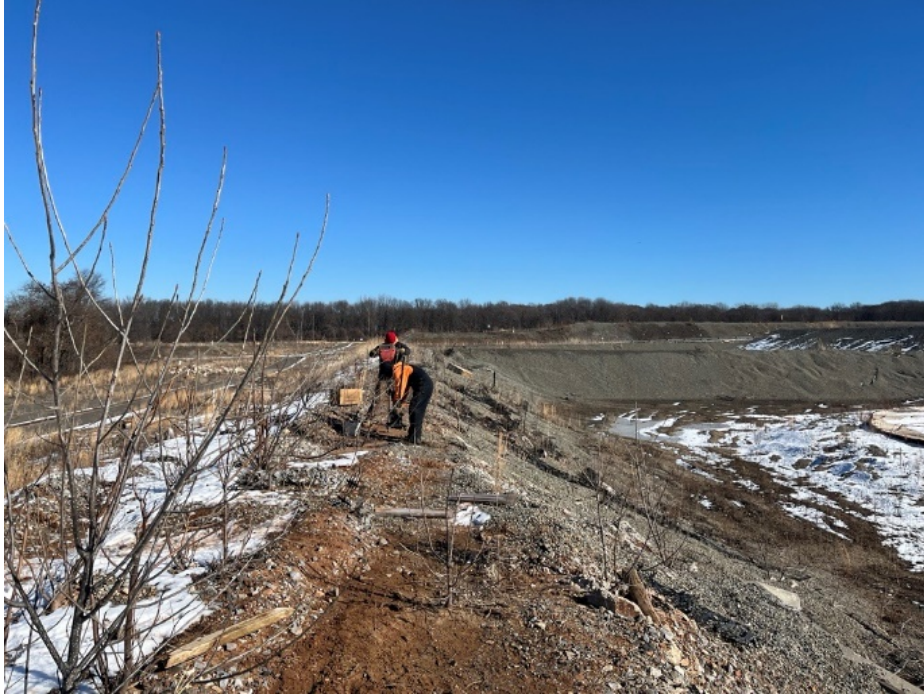
Photo 1: View of drilling activities in AST 16 berm, facing north.
