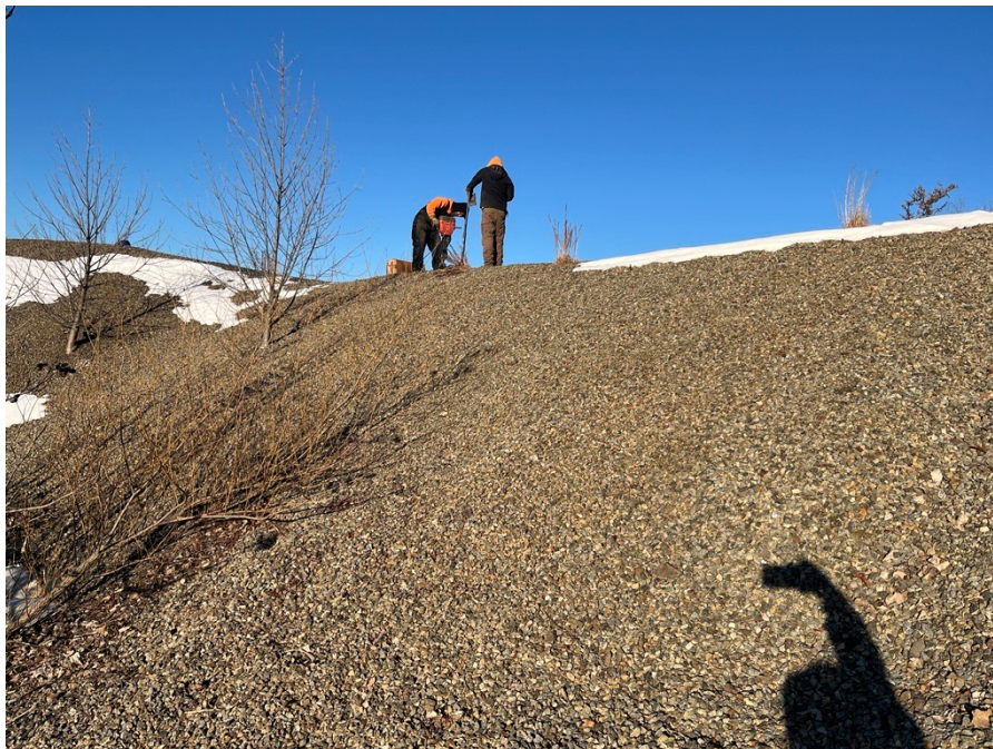
Photo 4: View of drilling activities in AST 16 berm, facing southwest.
