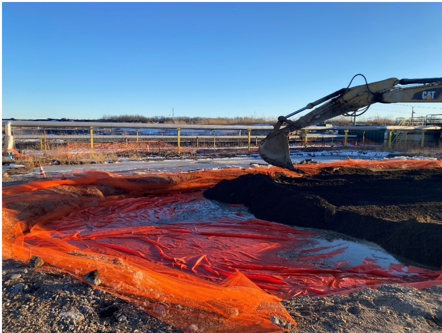
Photo 4: View of Exc. 5A geotextile layer and backfill activities, IRM 1 Eastern Area, facing east.
