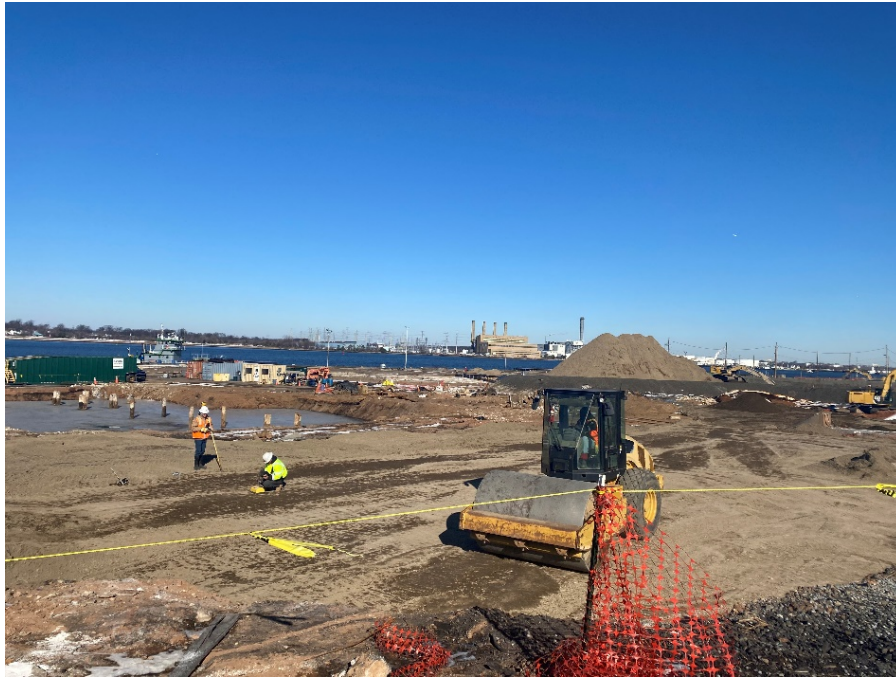
Photo 1: View of Exc. 9 backfill activities and compaction testing, IRM 1 Central Area, facing northwest
