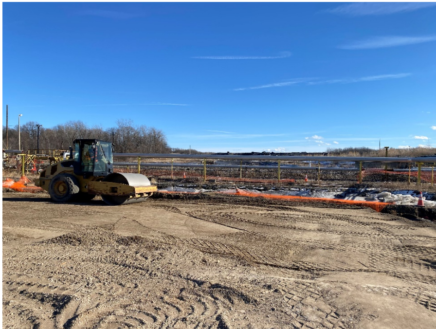
Photo 2: View of Exc. 5B compaction activities, IRM 1 Eastern Area, facing east.
