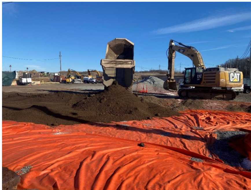
Photo 4: View of Exc. 1B backfill activities, IRM 1 Western Area, facing east.
