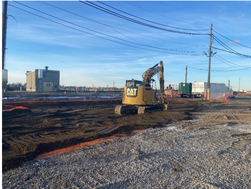
Photo 3: View of Exc. 1B backfill activities, IRM 1 Western Area, facing northwest.
