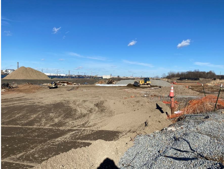
Photo 1: View of Exc. 9 backfill activities, IRM 1 Central Area, facing northwest
