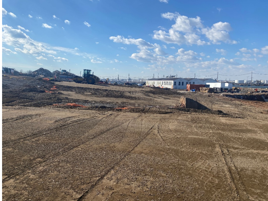
Photo 1: View of Exc. 9 compaction activities, IRM 1 Central Area, facing south.
