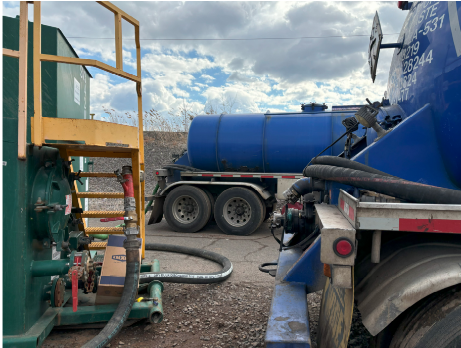
Photo 3: View of water filling activities, IRM 1 Eastern Area, facing south.
