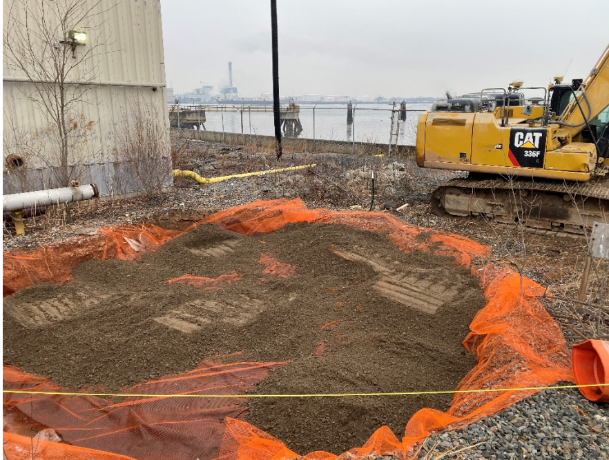
Photo 3: View of Exc 7, placement of geotextile layer, IRM 1 Eastern Area, facing north.
