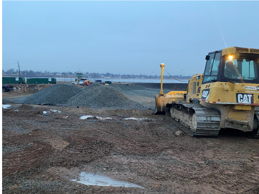
Photo 1: View of Exc. 9, Placement of top stone layer, IRM 1 Central Area, facing south.
