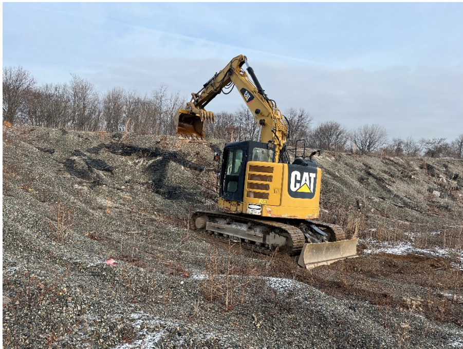
Photo 2: View of initial soil exposure along Berm 16, facing northwest.
