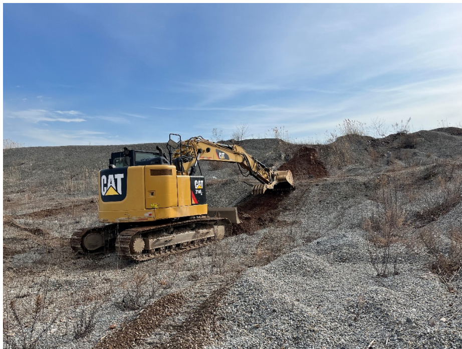
Photo 4: View of soil exposure with use of excavator bucket in Berm 16, facing south.
