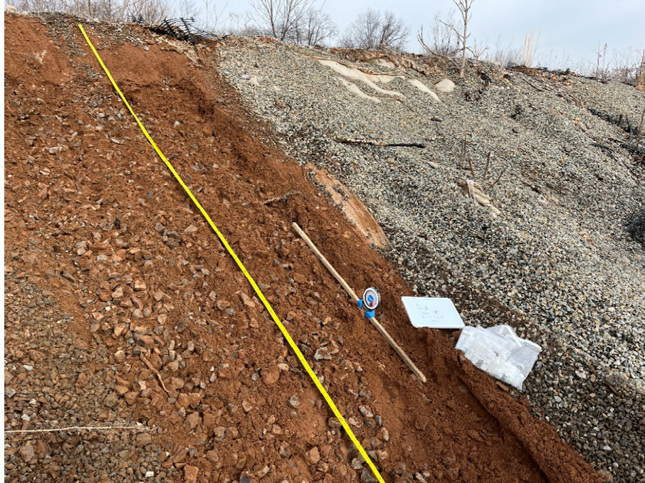
Photo 3: Screening of soils from Berm 16, facing north.
